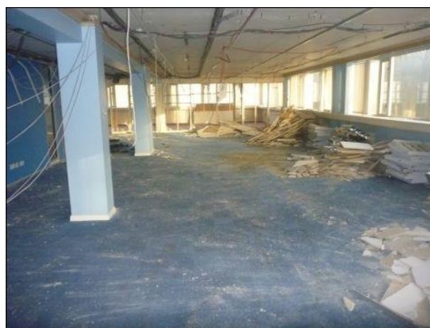
Photo 16: Building 1 internal area
