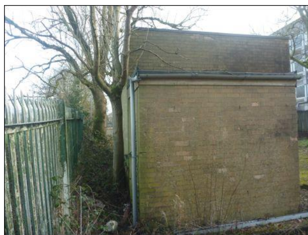
Photo 18: Building 2, western and northern elevations
