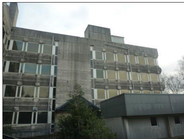
Photo 14: Building 1, western elevation, southern end
