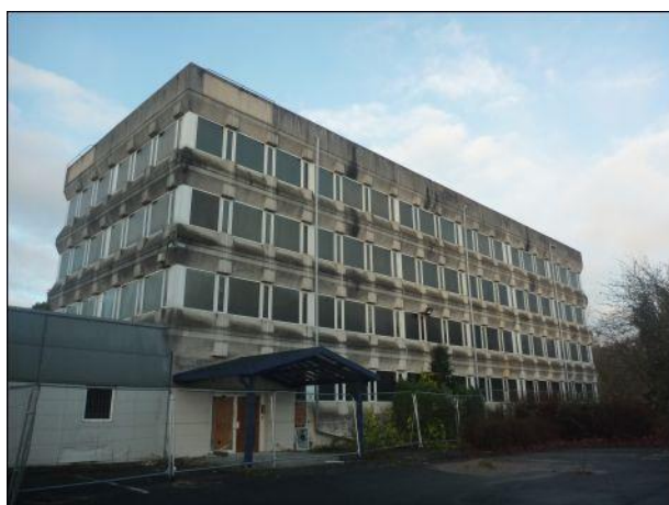
Photo 11: Building 1, eastern elevation
