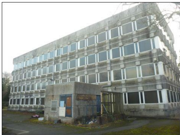
Photo 13: Building 1, northern elevation, western end and western elevation
