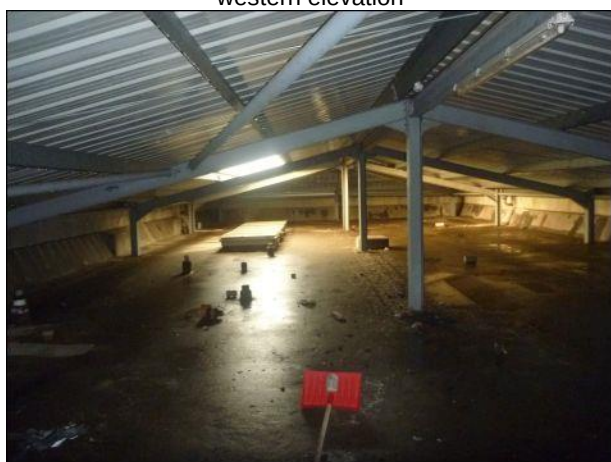
Photo 15: Building 1, roof void
