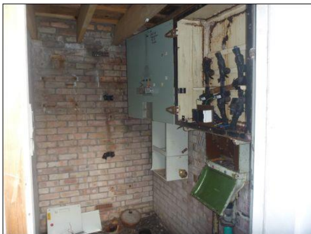
Photo 19: Building 2 internal area
