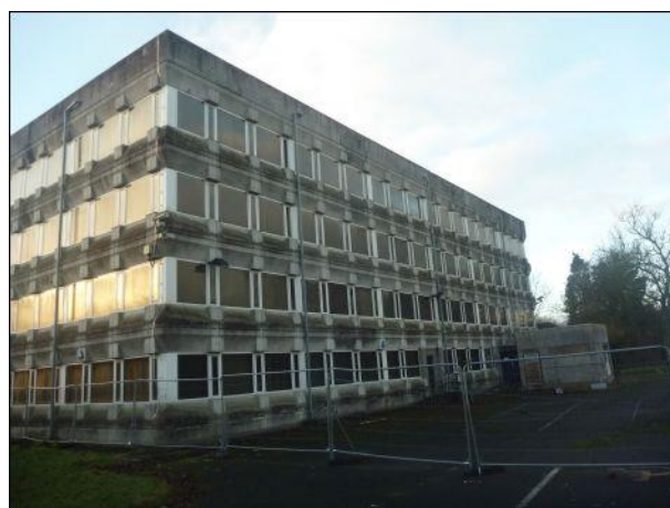
Photo 12: Building 1, northern elevation, eastern end
