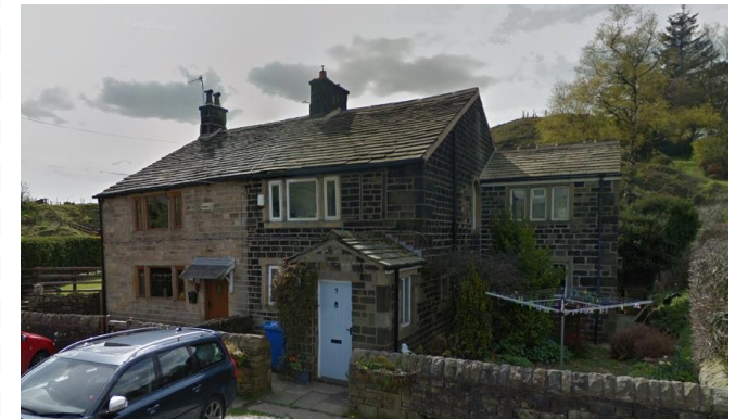
Semi Detached Cottages Salley Street / Calderbrook Road
