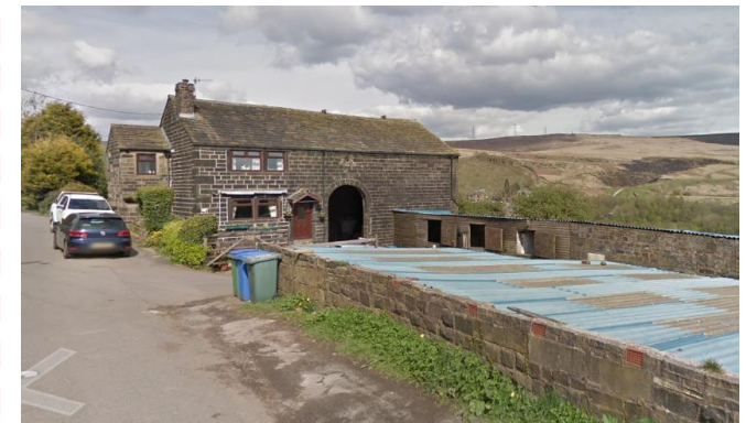
Farm House and Outbuildings Salley Street
