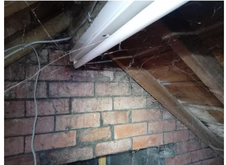
Photo 4: B1 – main loft void.
