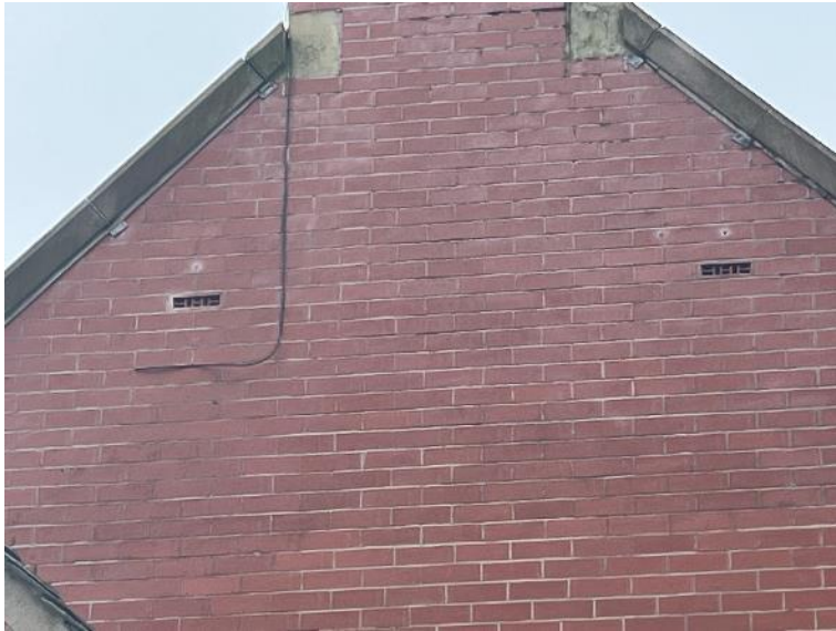
Photo 3: B1 – vents – northern elevation.
