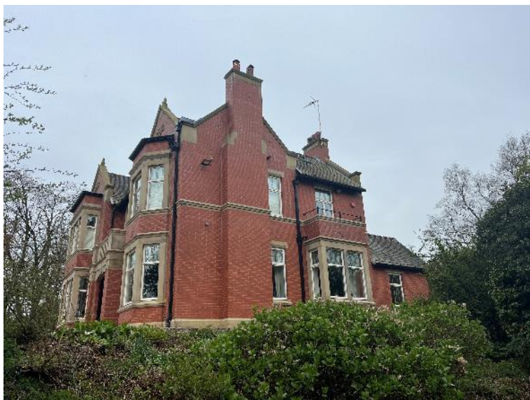
Photo 1: B1 – facing the eastern elevation.
