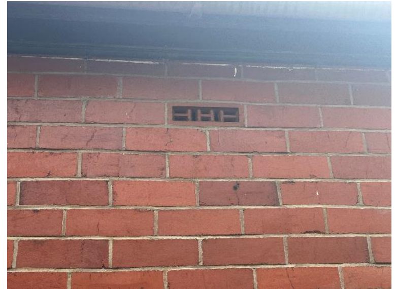
Photo 8: B2 – northern elevation vent.
