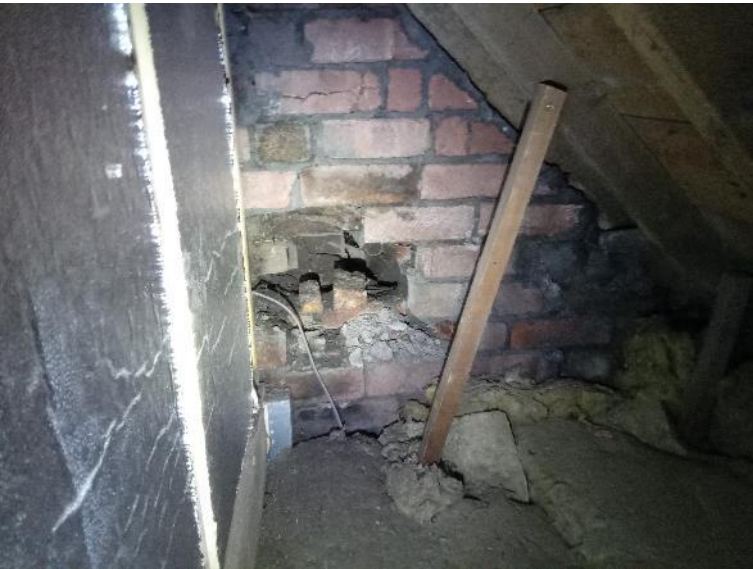
Photo 5: B1 - smaller loft void.
