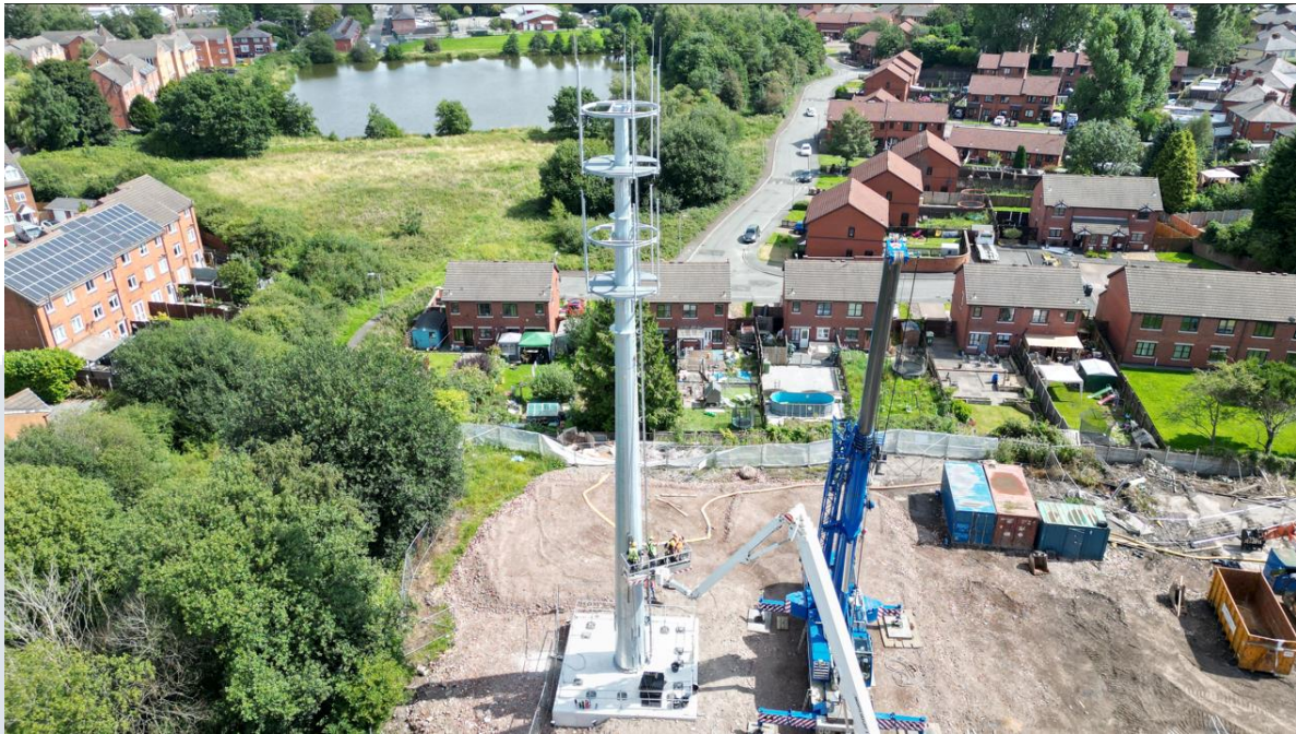
Figure 5 – Aerial imagery of a 30m-high tower deployed at Century Mill, George Street, Farnworth, BL4 9QW and approved by Bolton Council in 2022 (Source: Applicants drone imagery)
