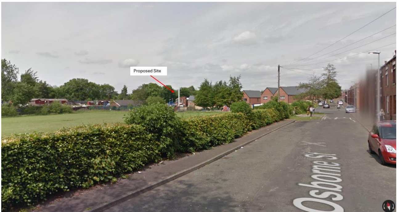
Figure 5: View of site from southwest on Osborne Street (Source: Google Street View, Mar 2023)
