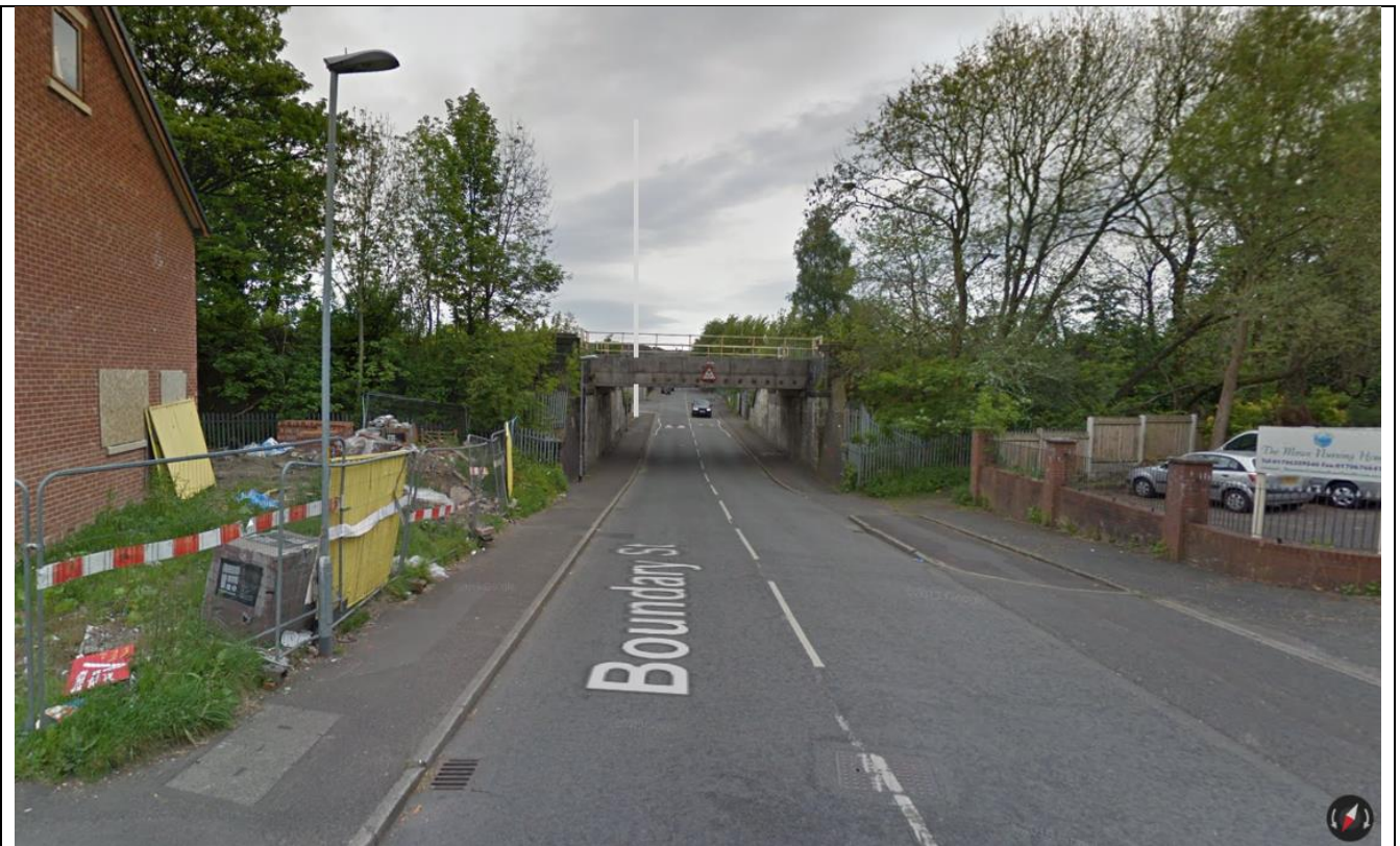
Figure 3: View of site from north beyond railway line (Source: Google Street View, 2019)
