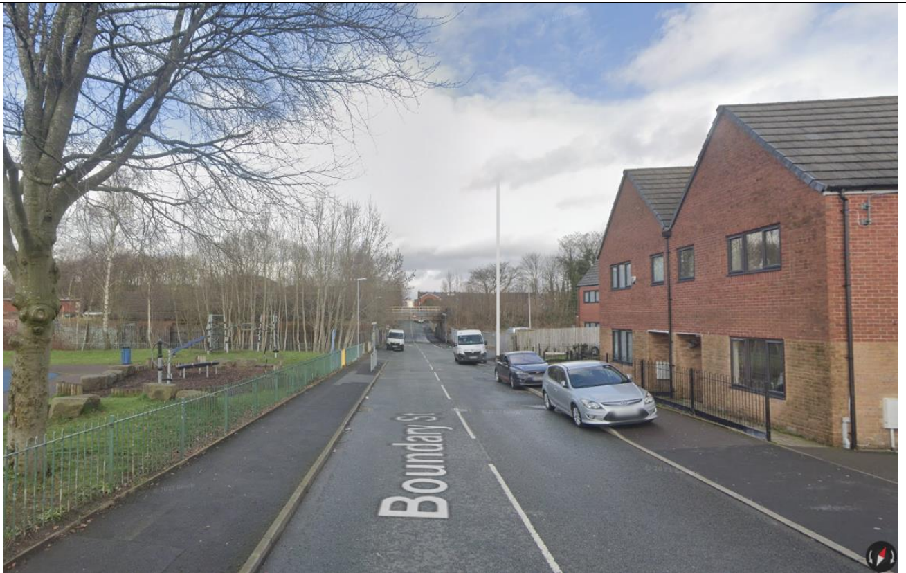
Figure 4: View of site from south (Source: Google Street View, Mar 2023)
