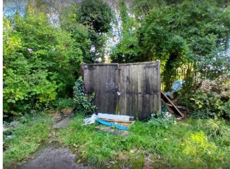
Figure 1 - Dilapidated shed located to the southeast of the site.
