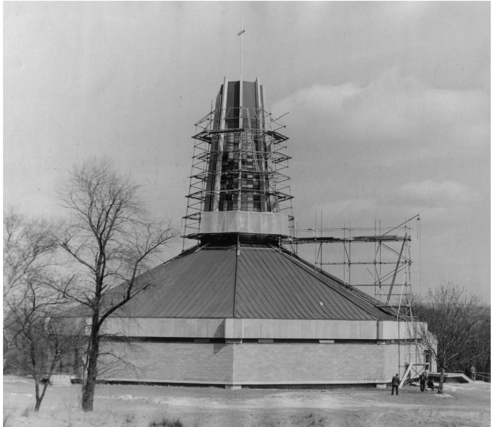
Figure 4.1 The Chapel during construction (Source: Rochdale Archives)
