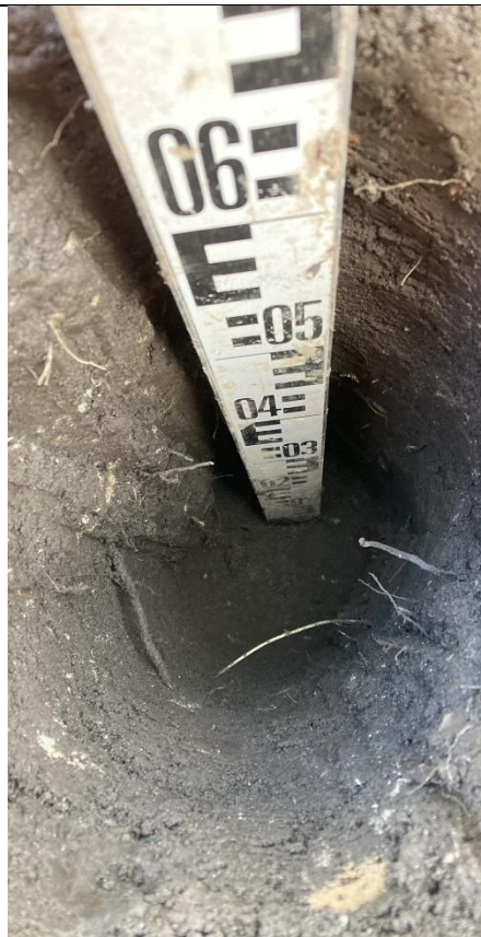
Plot 13: Internal View of excavation
