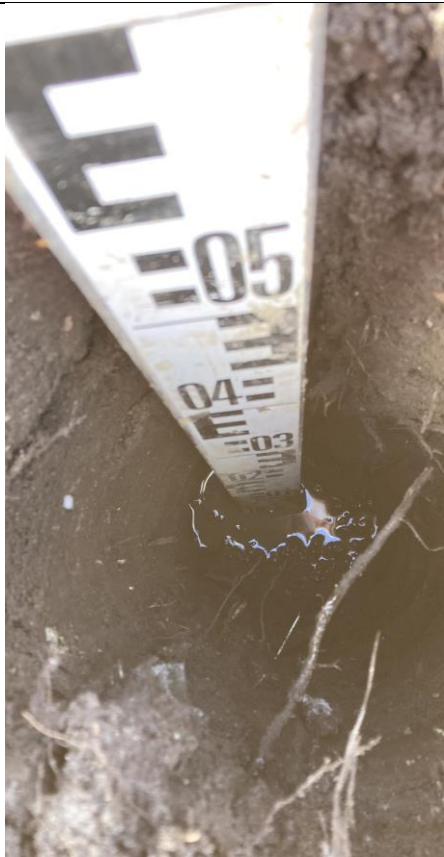
Plot 22: Internal View of excavation
