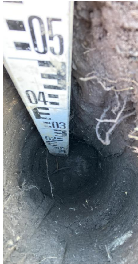
Plot 10: Internal View of excavation
