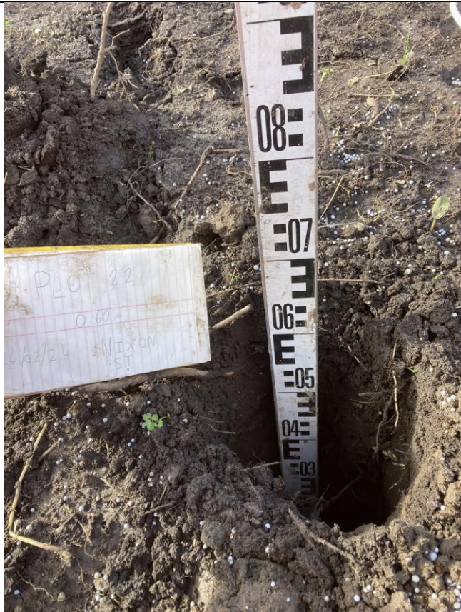
Plot 22: Overview of excavation
