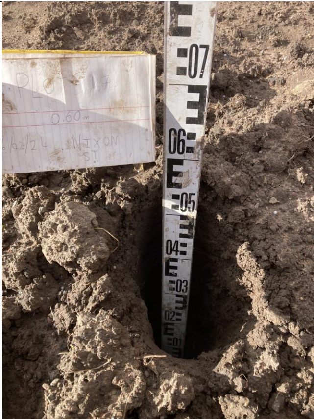
Plot 17: Overview of excavation
