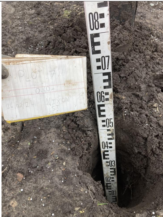
Plot 7: Overview of excavation
