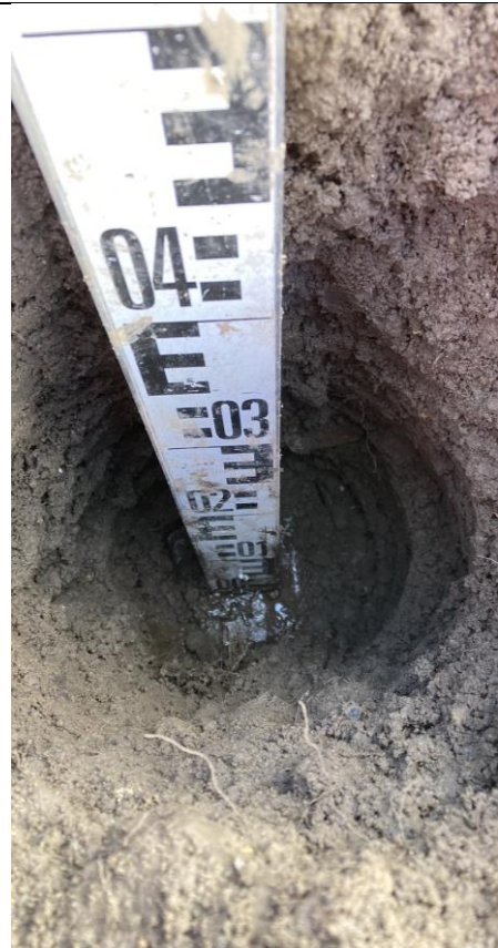
Plot 14: Internal View of excavation
