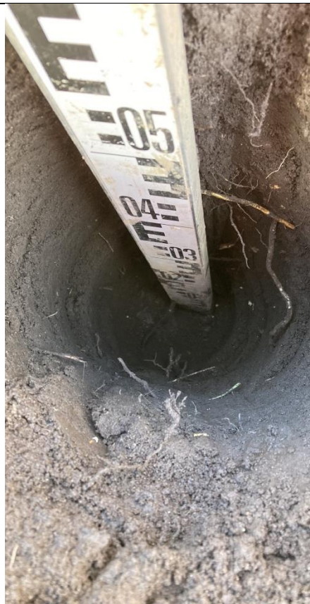
Plot 11: Internal View of excavation
