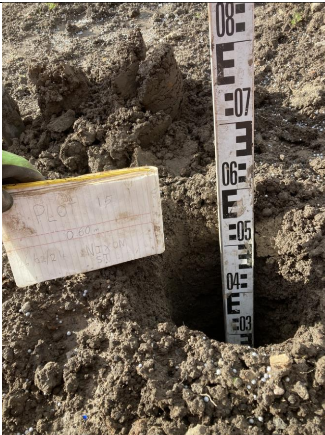
Plot 15: Overview of excavation
