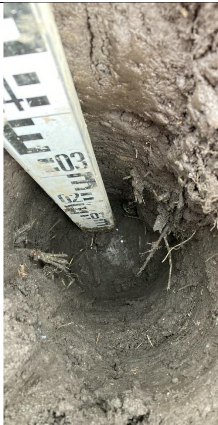
Plot 7: Internal View of excavation
