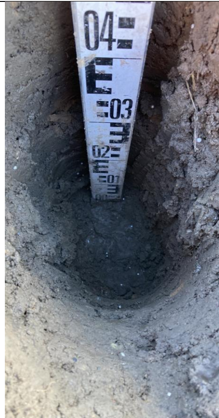
Plot 19: Internal View of excavation
