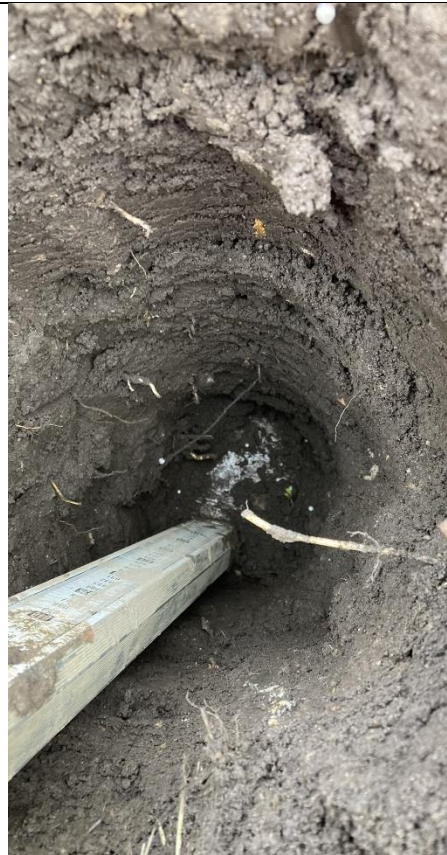
Plot 6: Internal View of excavation
