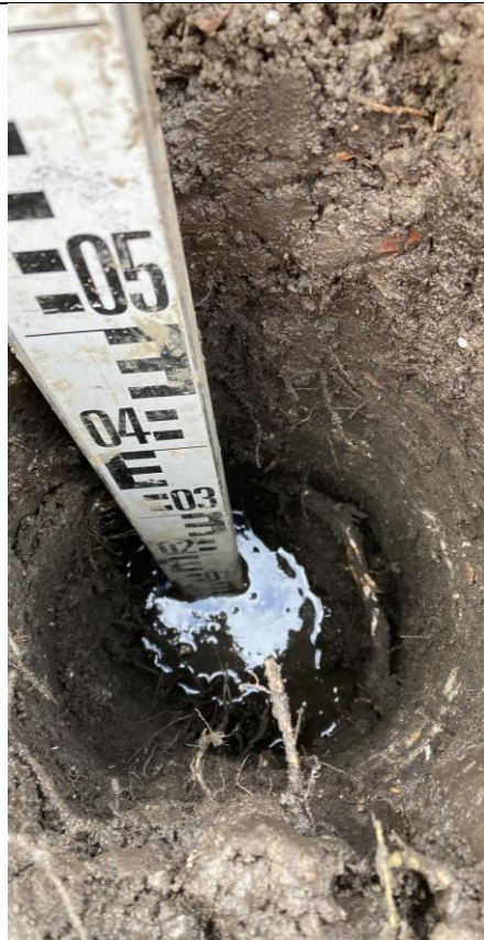
Plot 23: Internal View of excavation
