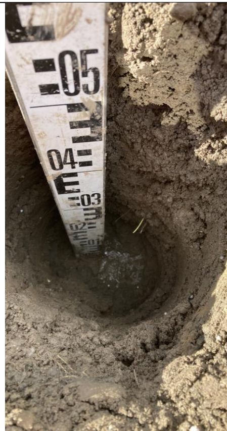
Plot 15: Internal View of excavation
