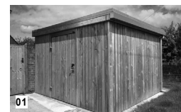
01 WASTE MANAGEMENT STORE Concrete base with 2.4m high timber palisade fencing with galvanized structure and green roof.
