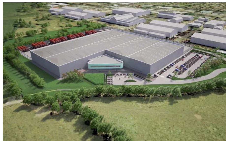
PORTAL MILL, MELKSHAM
