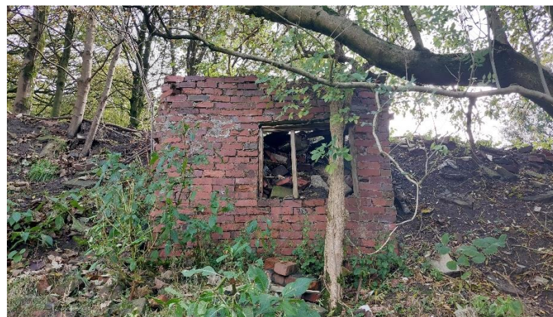
Photograph 8: Derelict building on the site's northern boundary. Building was of negligible suitability to support bats.
