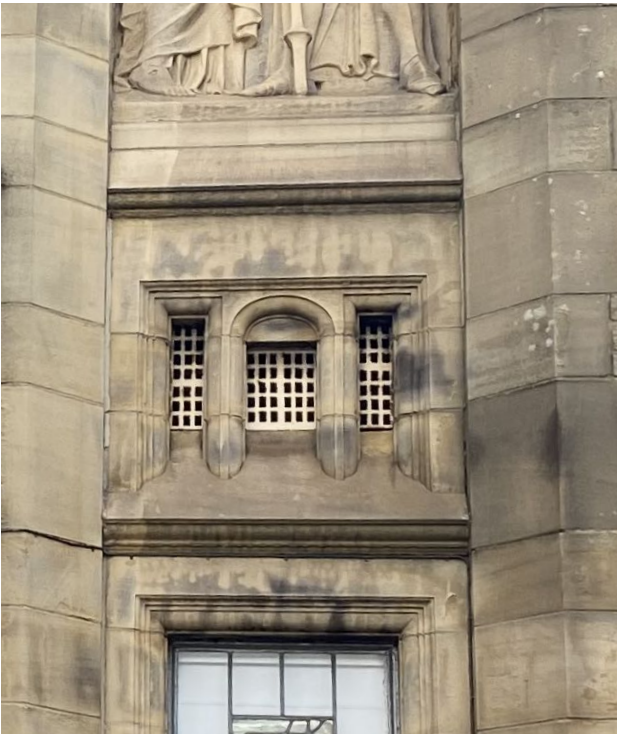
Image 04/04 - External photograph looking at a typical ventilation grille condition.
