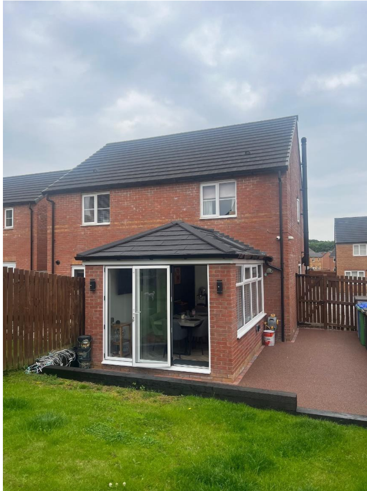
Orangery to the rear elevation of No. 8 Stubbs Road
