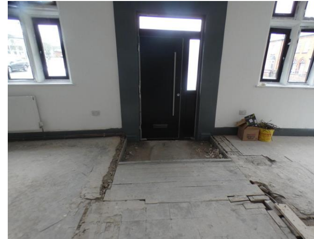
View of external door with step up to floor level
