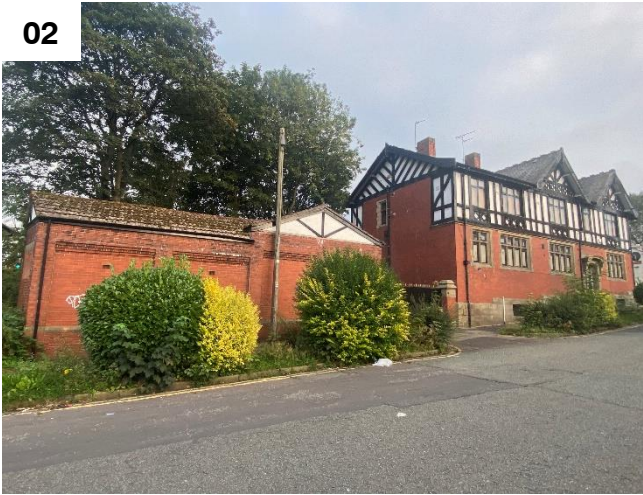
View of existing building and garage from Manchester Road
