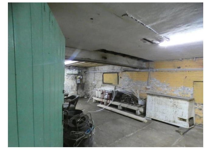
View of basement store room 4
