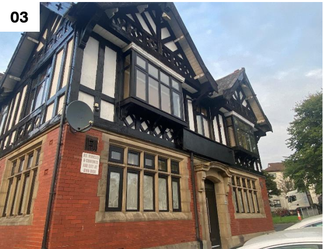
View of existing building from car park
