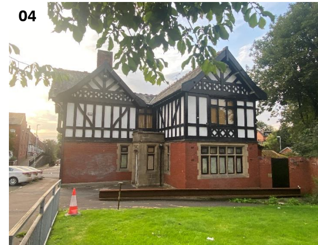
View of existing building from grass verge to the east
