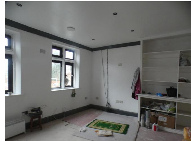
View of the existing living room on the first floor
