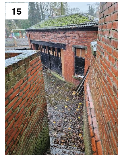
View of existing garage from external stairs
