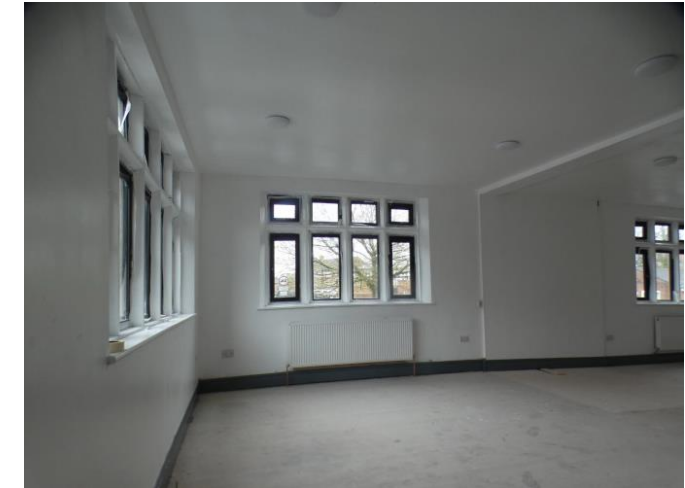
View of existing windows in main open space area
