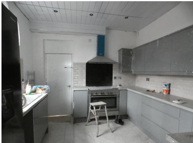
View of the existing kitchen renovation on the first floor
