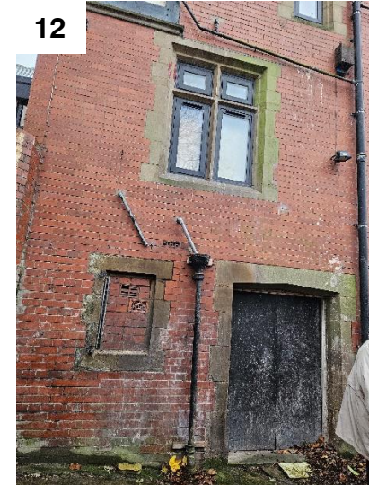
View of existing basement door
