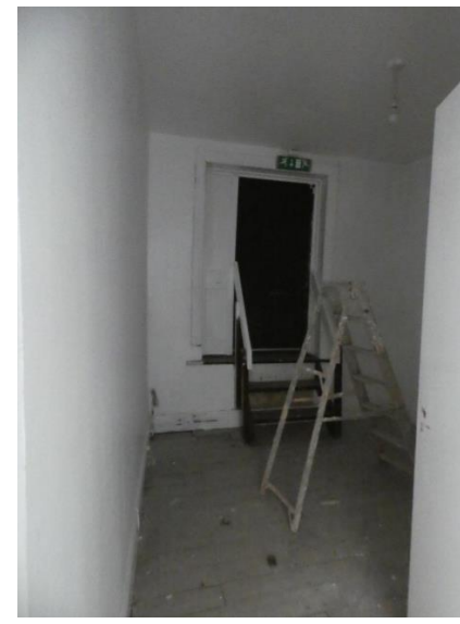
View of fire escape door on the first floor
