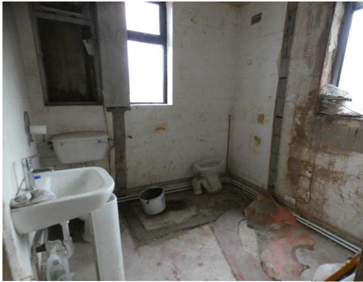
View of toilets located in one-storey extension 1
