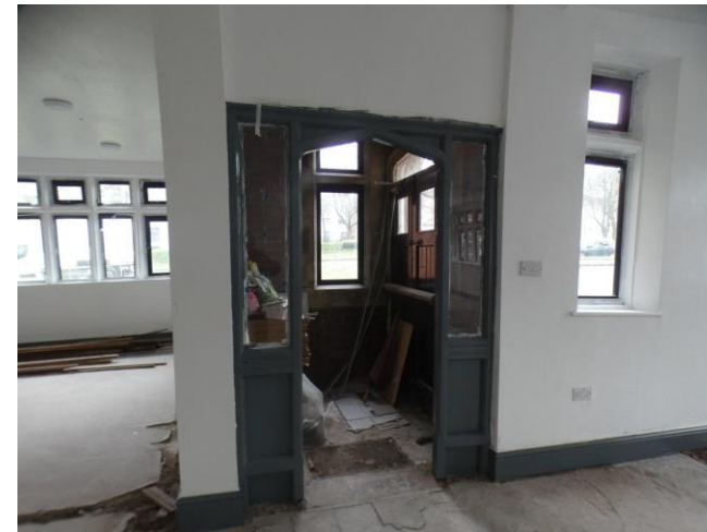
View of Internal door and porch area
