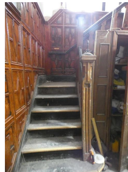
View of the bottom of existing staircase
