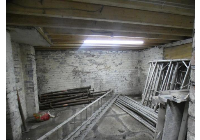
View of basement store room 2
