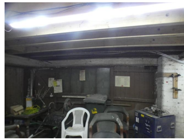
View of basement store room 3
