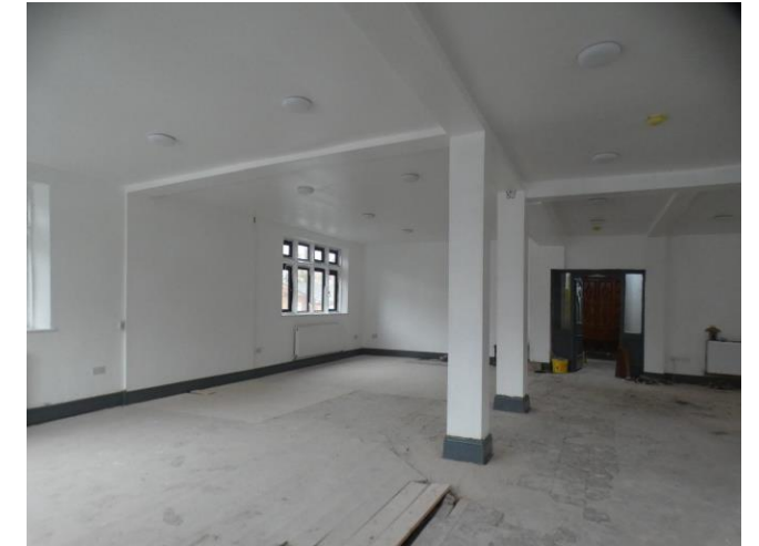
View of existing columns supporting the existing structure
