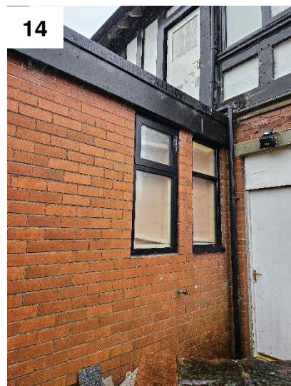
View of existing one-storey extension
