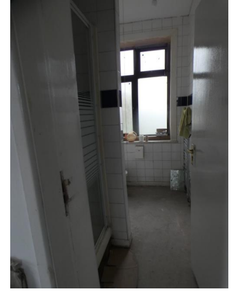
View of bathroom refurbishment on first floor
