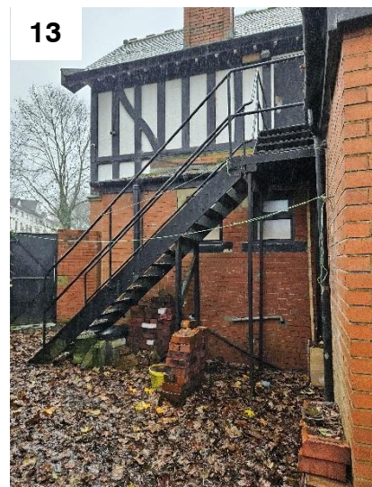
View of existing fire escape and extension
