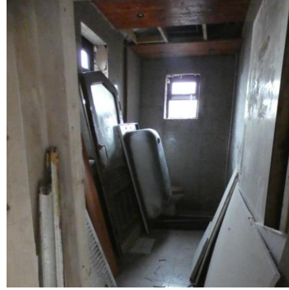
View of toilets located in one-storey extension 2
