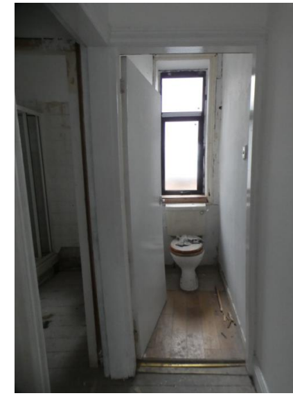
View of w/c partially refurbished on first floor
