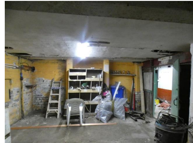
View of basement store room 1
