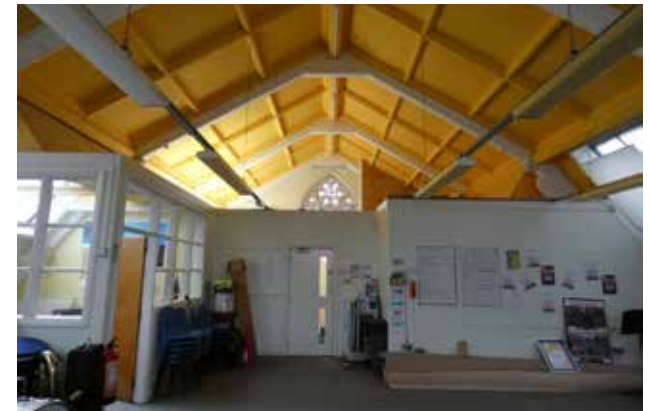
Modern partitions and mezzanine removed to reveal Bright Hall
