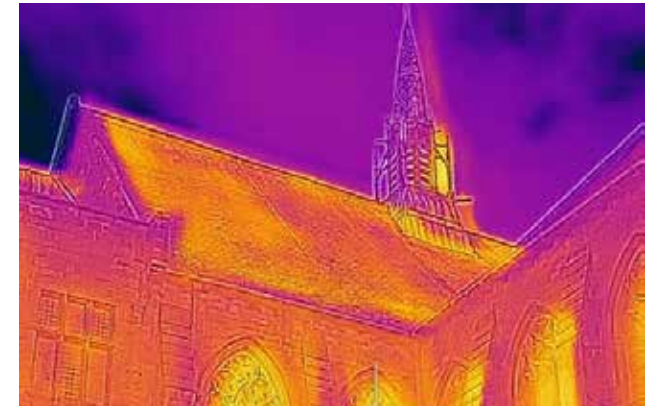
Overall it is clear that the glazing in general is the big area of heat loss.
