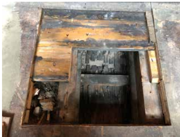
Opening up works
