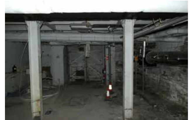
Basement to undergo stripping out and structural works
