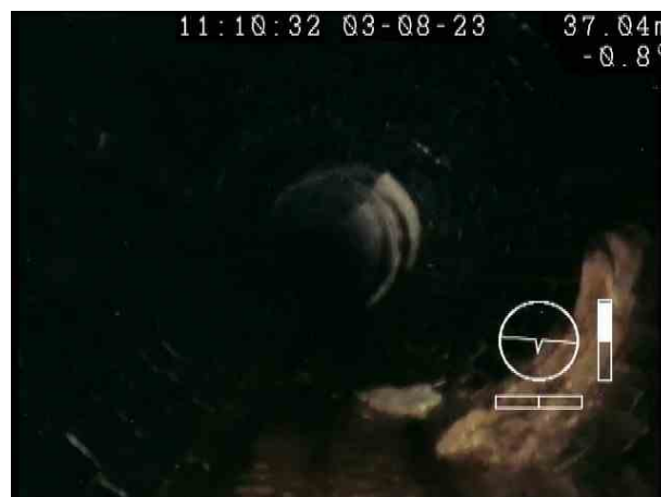
MH2X_ed12cab5-166a-4e04-9059-7607abf8a7c8_20230807_143902_719.jpg, 00:02:51, 37.04 m Connection other than junction at 03 o'clock, 225mm dia
