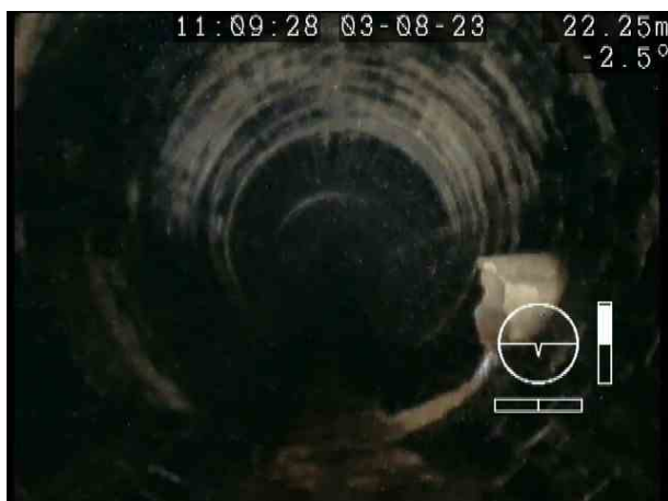
MH2X_0ce11f09-7e93-46ff-b017-77710b23b2b6_20230807_143823_705.jpg, 00:01:46, 22.25 m Connection other than junction at 02 o'clock, 255mm dia
