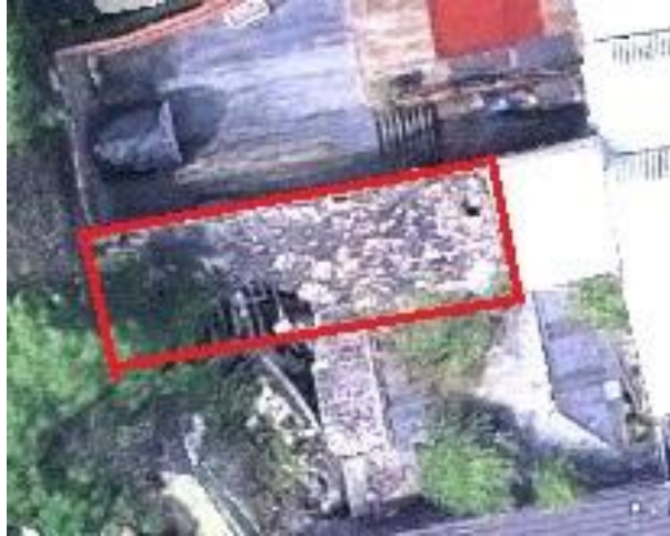
Aerial view of roof of brick building
