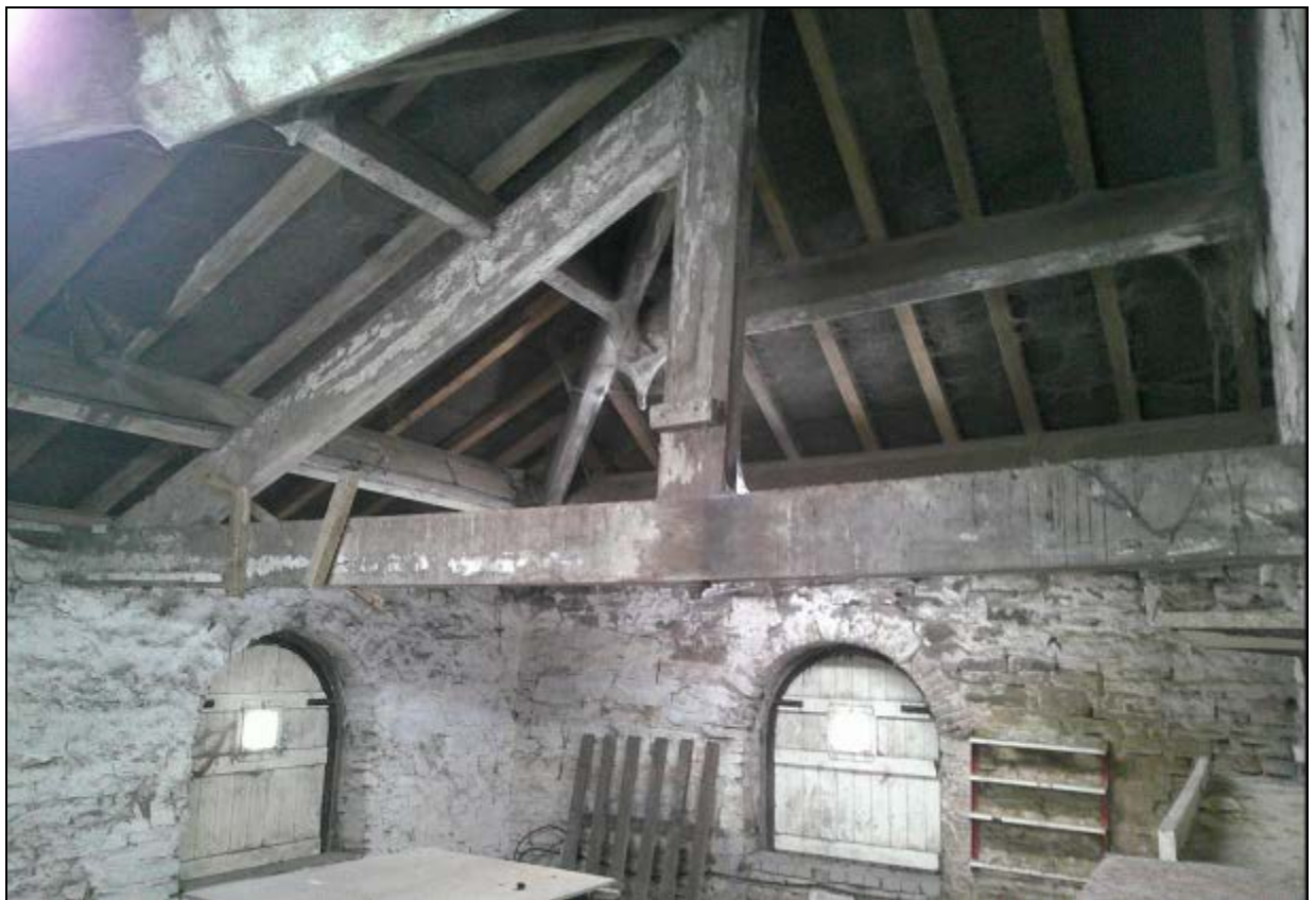
16. Half truss in loft over western shippon
