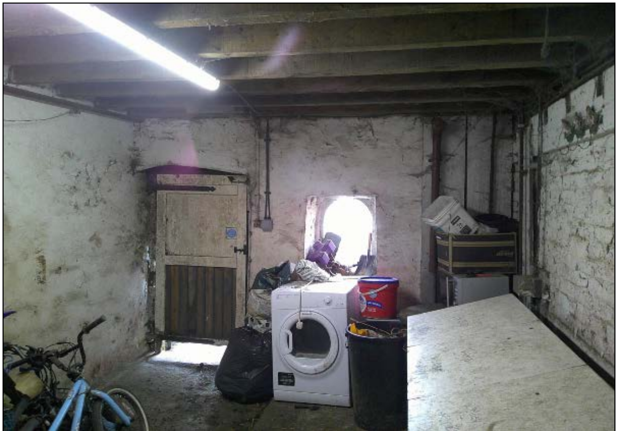
12. Interior of the shippon
