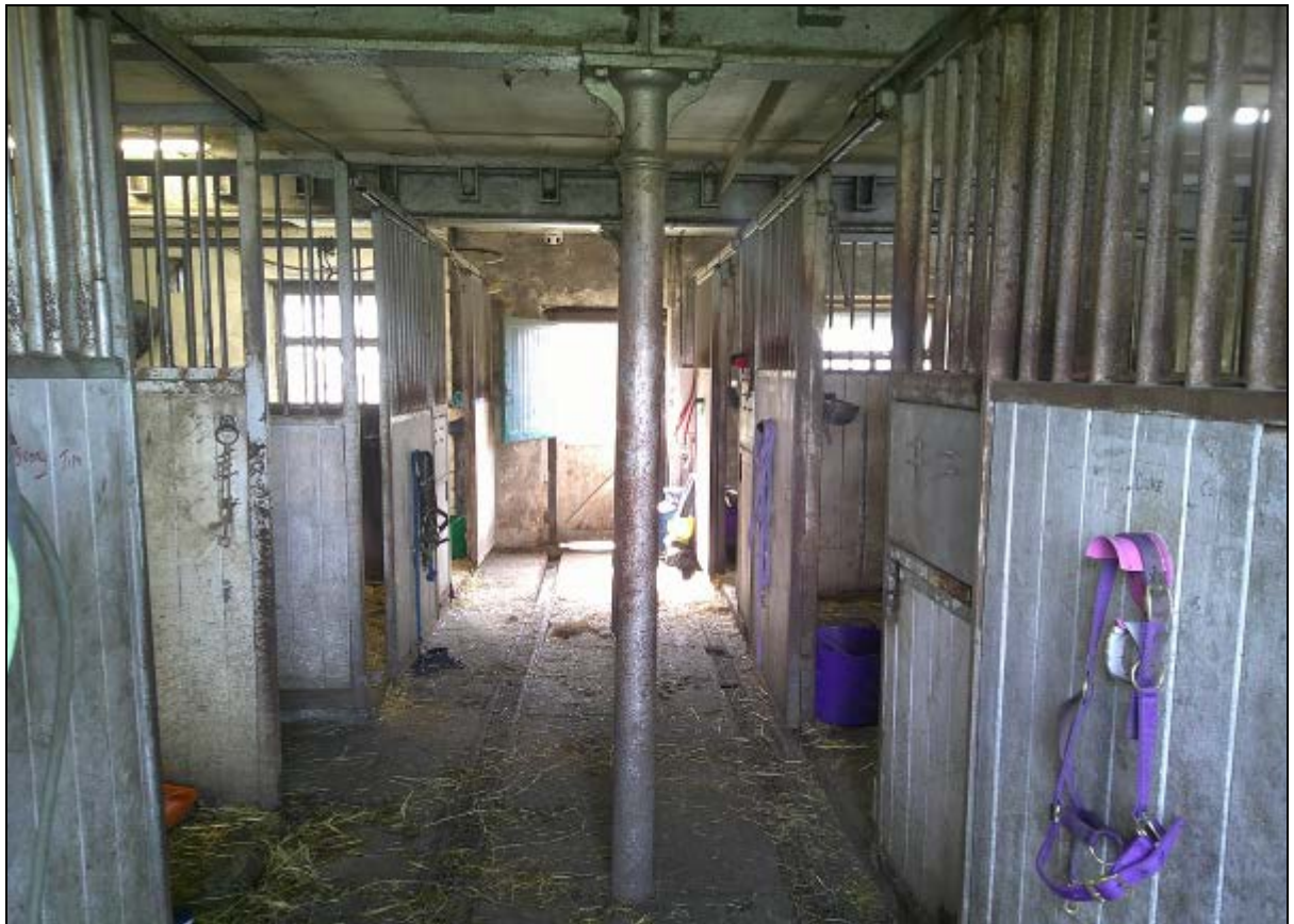
13. Through-passage of stables, with later, ex-situ, steel columns
