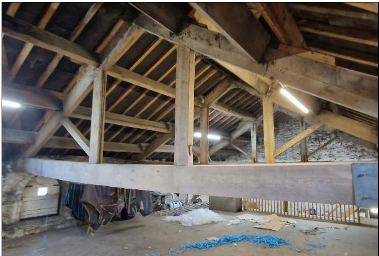
14. Roof trusses over stables are not the original
