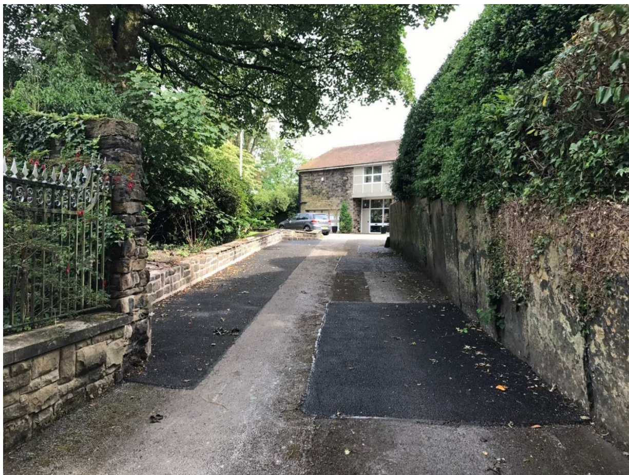
Figure 2.1 – Widened Access Driveway
