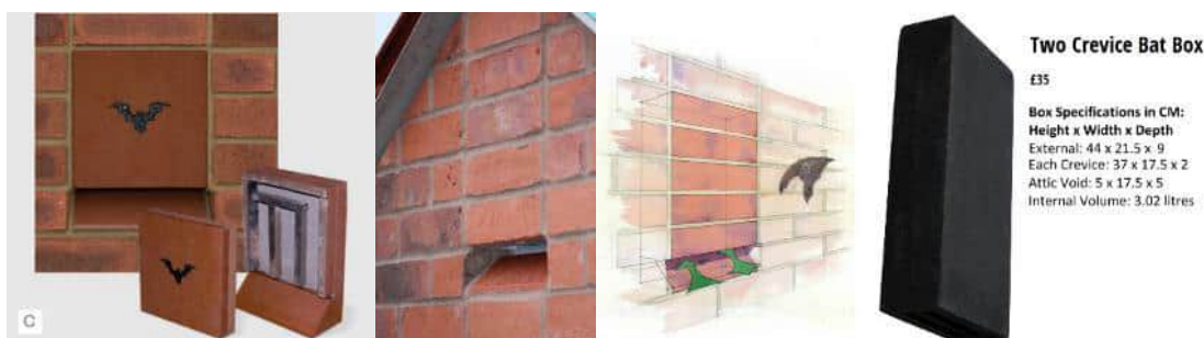
Insert 1: Examples of integrated bat access panels and an externally mounted box 7
