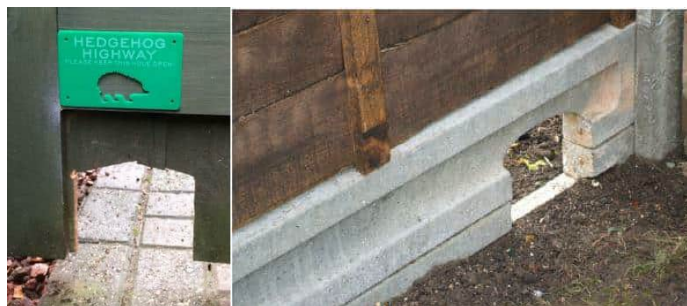
Insert 3: Showing wildlife access gap within fencing
