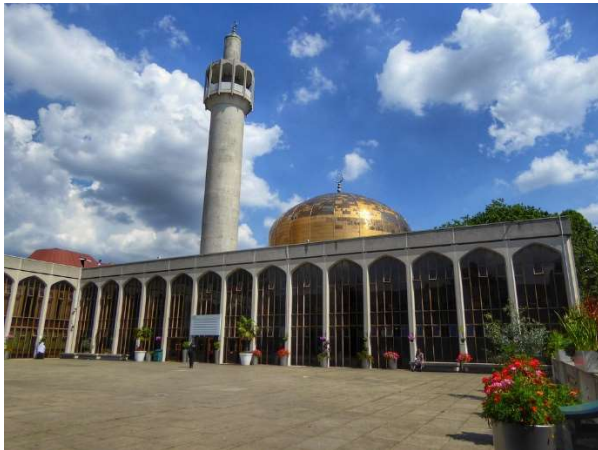
Figure 3.21 External photograph of the London Central Mosque (Source: www.bing.com , accessed 13/09/24).
