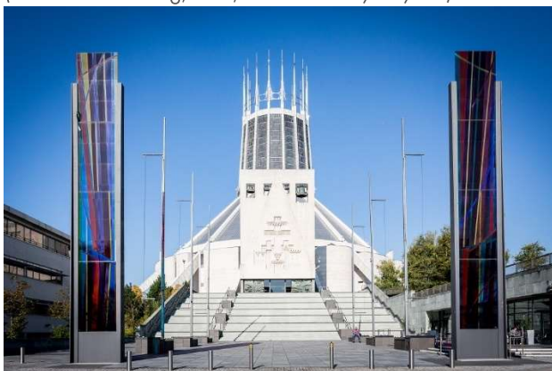
Figure 3.23 External photograph of the Liverpool Metropolitan Cathedral (Source: www.placenorthwest.co.uk , accessed 13/09/24).
