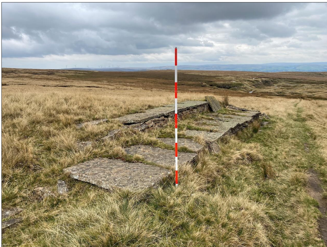
Plate 28: Sandstone construction (Asset 1152) probably associated with former tramway (right of frame), northwest of Ding Quarry, viewed from the northwest.
