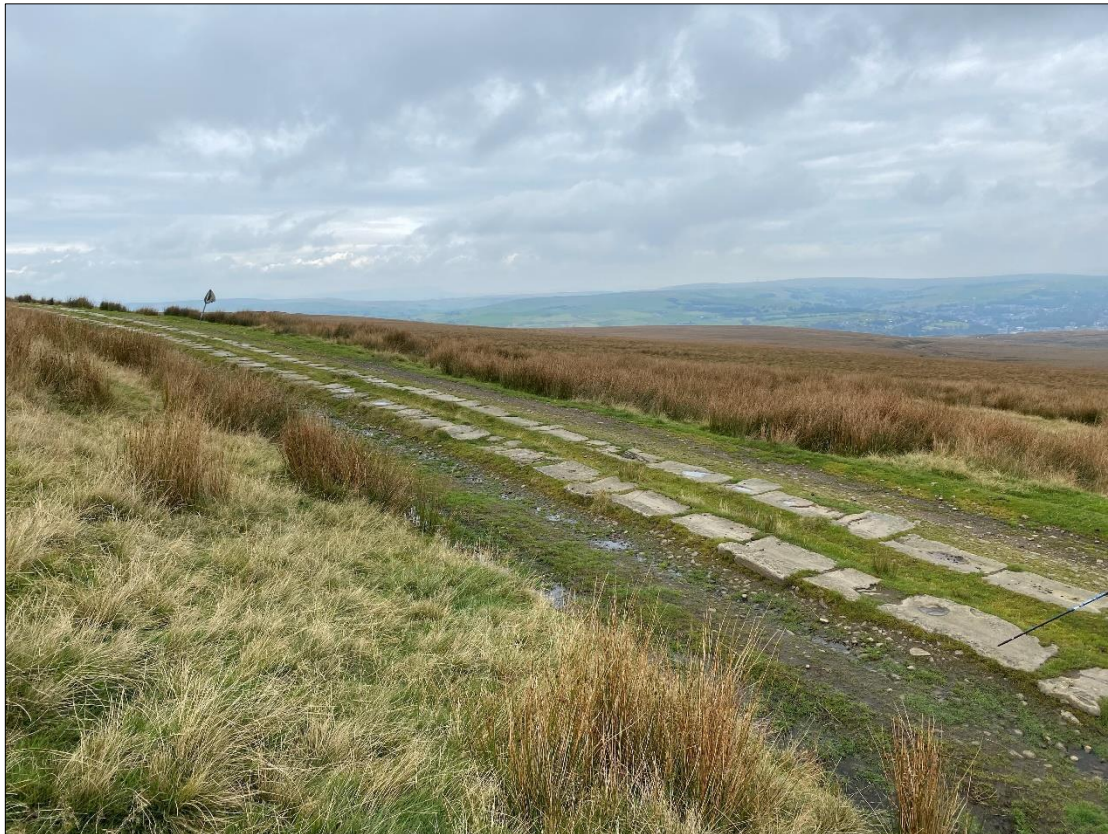
Plate 19: Looking northeast across a section of Rooley Moor Road (Asset 828) at Top of Leach.
