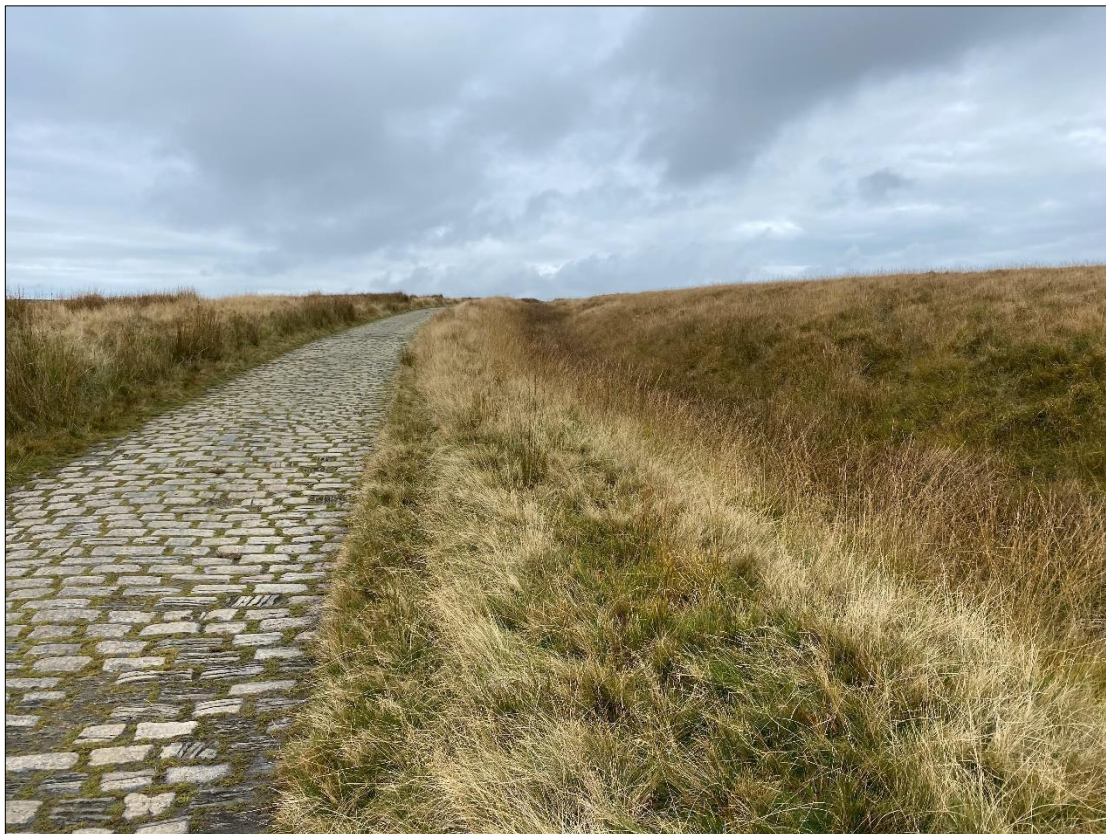
Plate 17: Looking north along a section of Rooley Moor Road (Asset 828) at Hamer Hill.
