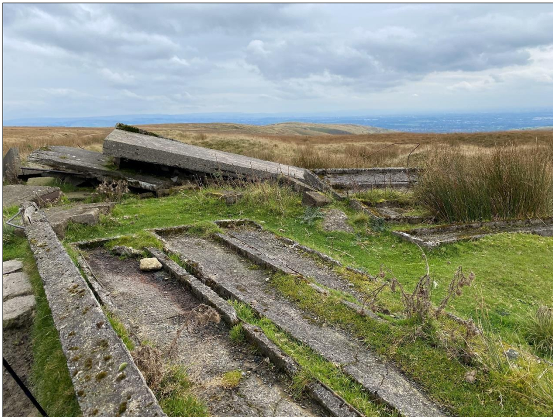
Plate 29: Structural remains alongside the track above (northeast of) Ding Quarry, looking southeast.
