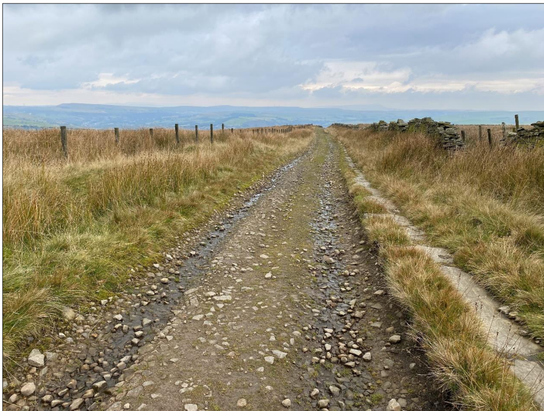
Plate 20: Looking NNW along a section of Rooley Moor Road (Asset 828) crossing Brandwood Moor.
