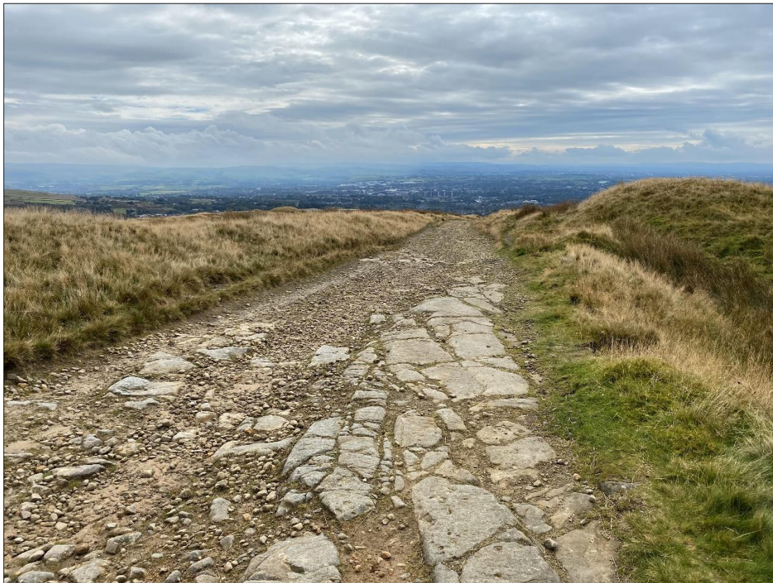
Plate 16: Looking southeast along a section of Rooley Moor Road (Asset 828) at Pike Brow.
