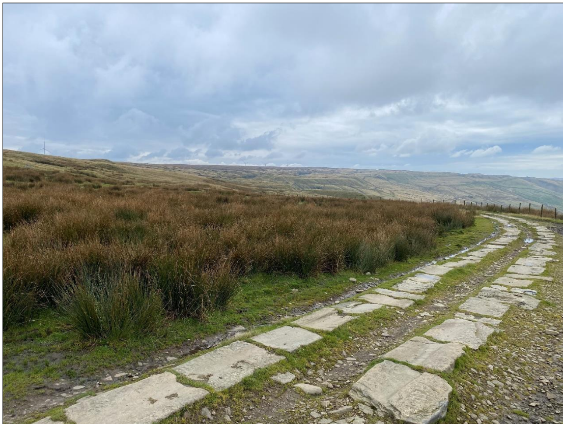
Plate 27: Looking east along the former tramway (a branch of Asset 189), now a footpath, at the eastern end of Cragg Quarry, close to its junction with Rooley Moor Road.
