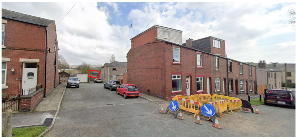
The nearest residential properties on Duke Street with existing double height garage highlighted in background.
