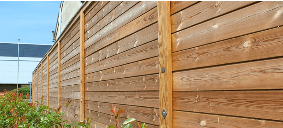
Timber fencing (ref 11)
