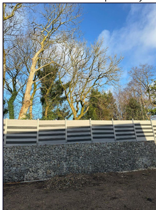
Figure 2. Installation of wall within RPA of third-party trees
