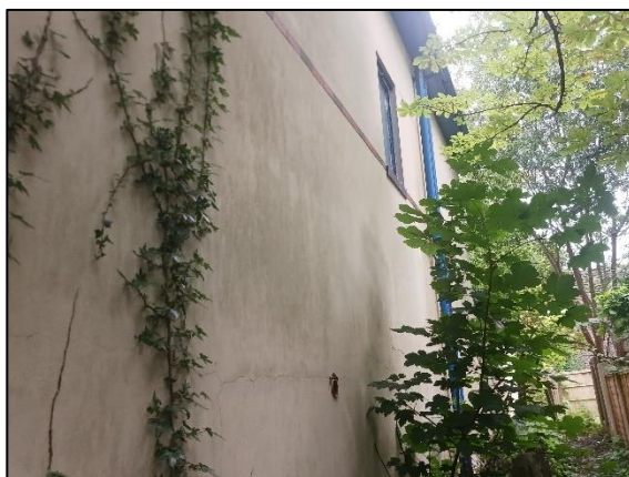
Figure 2.4: View along the north side of the building.
