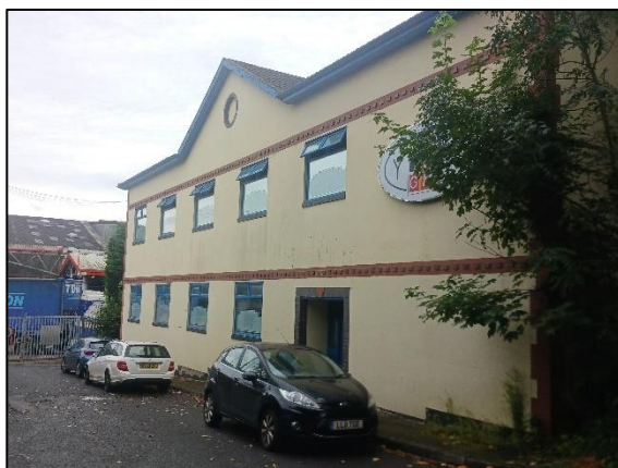
Figure 2.2: View of the east elevation of the building (Cheetham Street).
