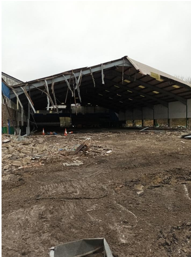
Plate No: 11. Demolition works of main arena
