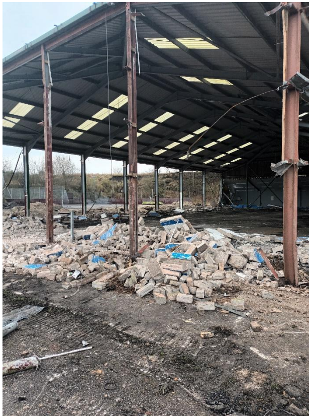
Plate No: 12. Demolition of smaller indoor pitch
