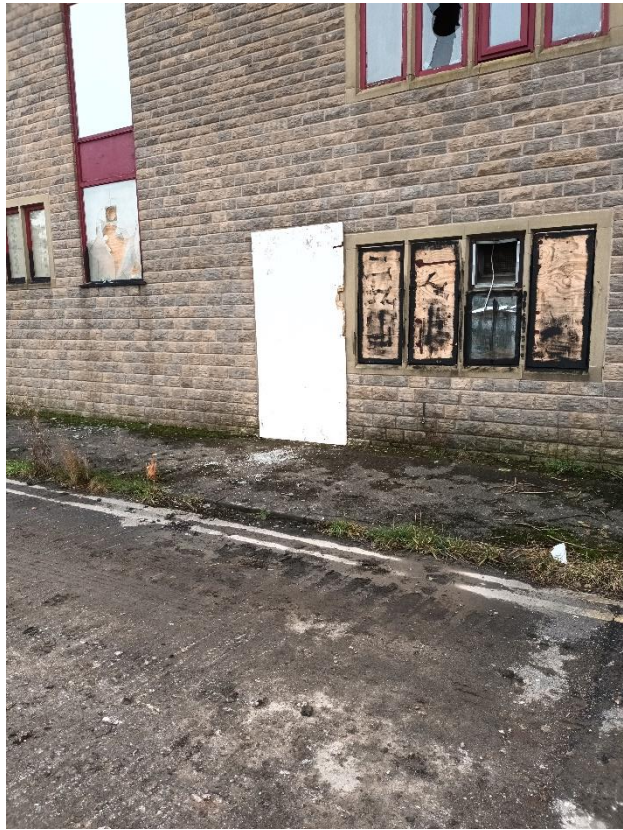
Plate No: 13. Site security of brick structure
