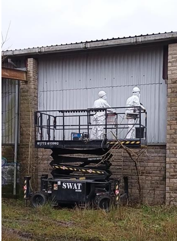
06/03/2018 Plate No: 4. Removal of asbestos sheeting
