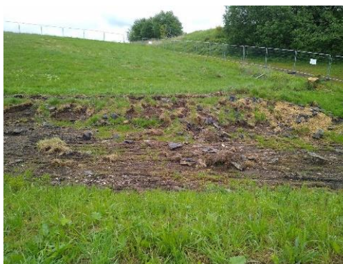
Photograph 4: Stones not removed after the dismantling of the stone wall.
