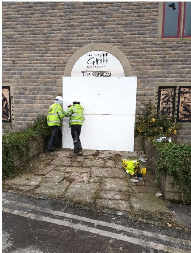
Plate No: 14. Site security of brick structure
