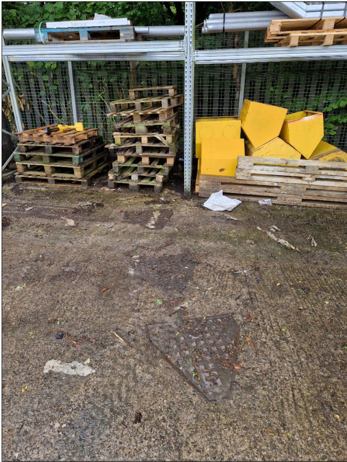
Petrol Interceptor Location View
