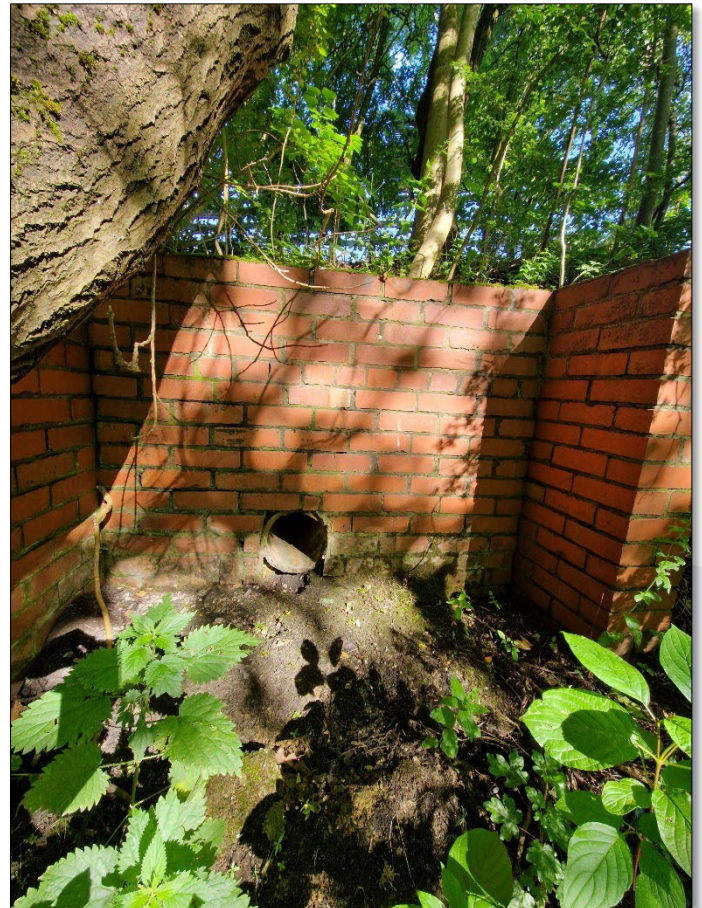
Pond Inlet Headwall
