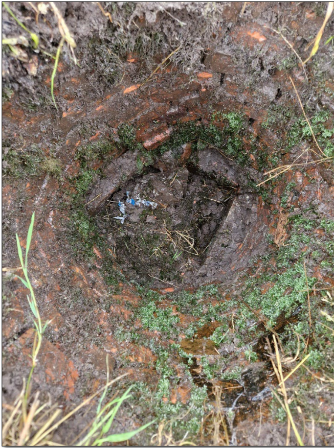
MH3 Internal View During Clearing
