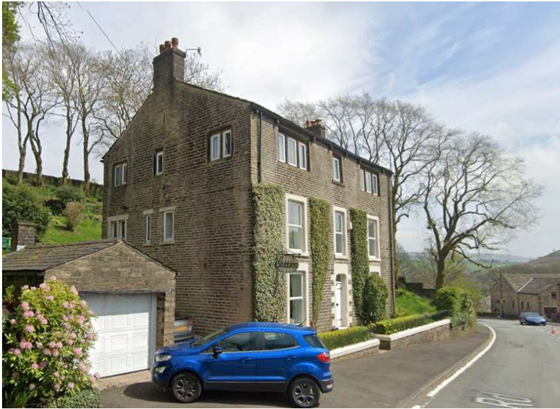
Denshaw Road – A legible fenestration arrangement along the front façade (Google Maps)
