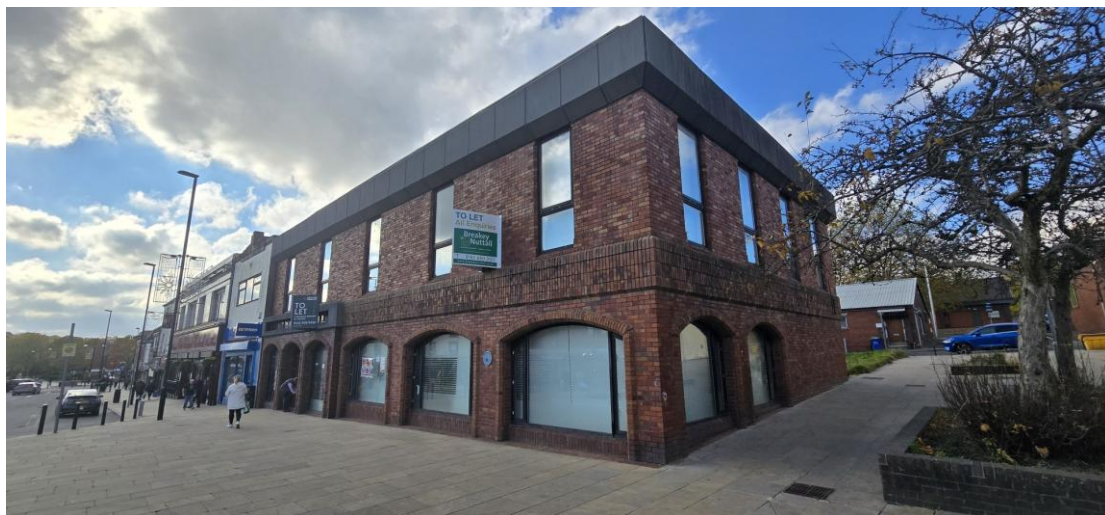
View of the existing vacant bank building.
