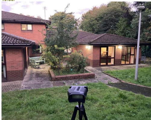
Photograph G: Western elevations; photo taken at approximately 19:30.
