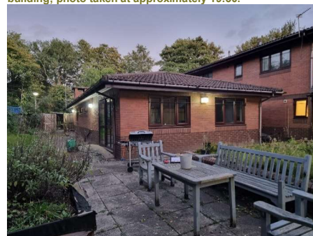
Photograph D: South-eastern section of building; photo taken at approximately 20:00.
