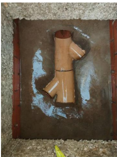
SWMH1 POST CLEAN
