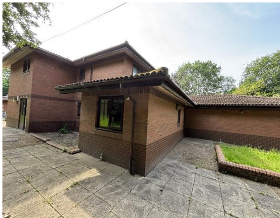
Single storey masonry wall supporting timber trussed roof
