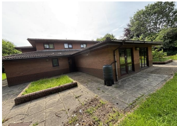
Single storey masonry wall supporting timber trussed roof
