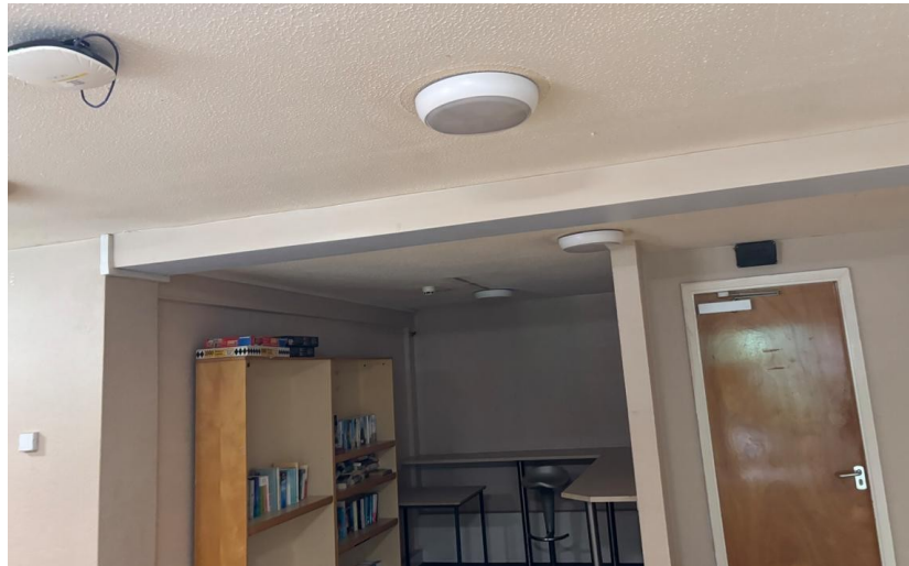
Steel beam supported by internal walls
