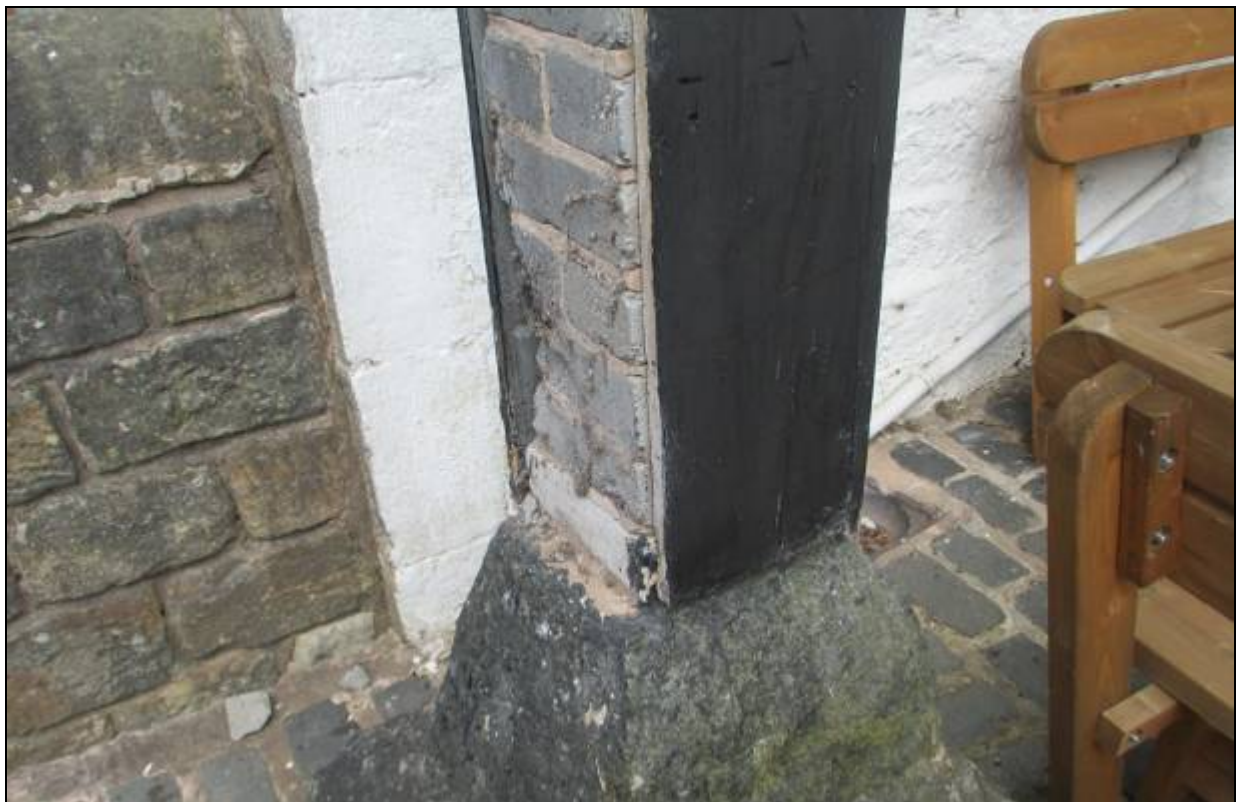
13. Boxed-in stock brick pillar supporting the steel beam
