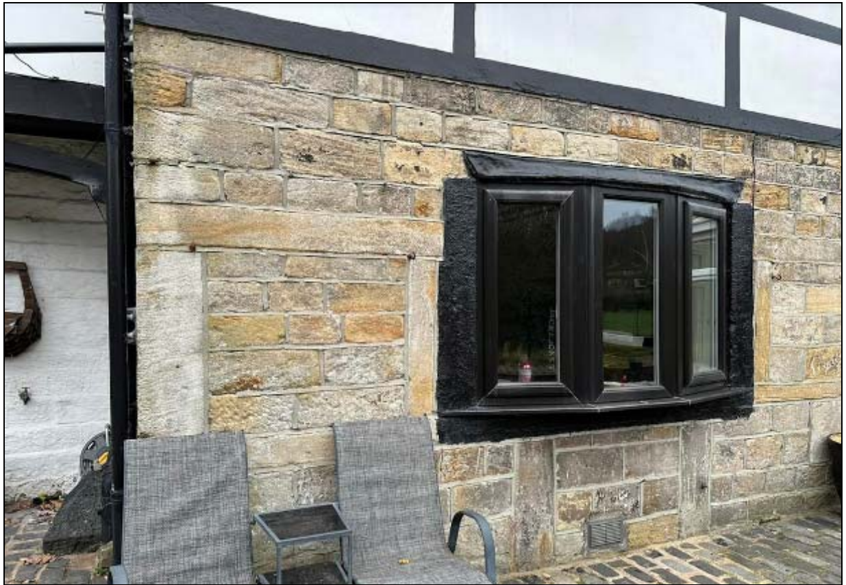
7. Ground floor central window seems to have replaced doorway; blocked window to its right
