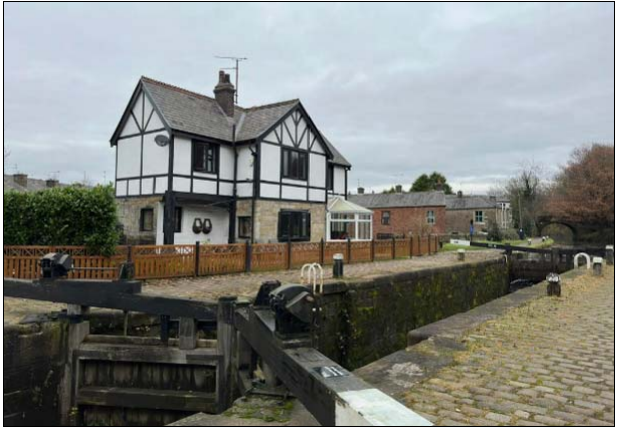
1. The Lock House, viewed from across Lock 48
