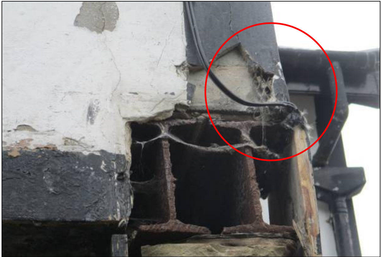
14. Outer wall above the steel beams is also stock brick
