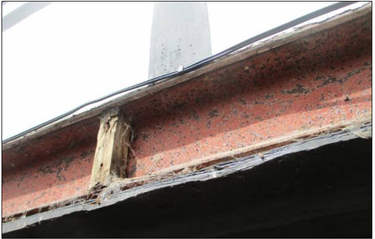
12. Steel beam supporting the jetty
