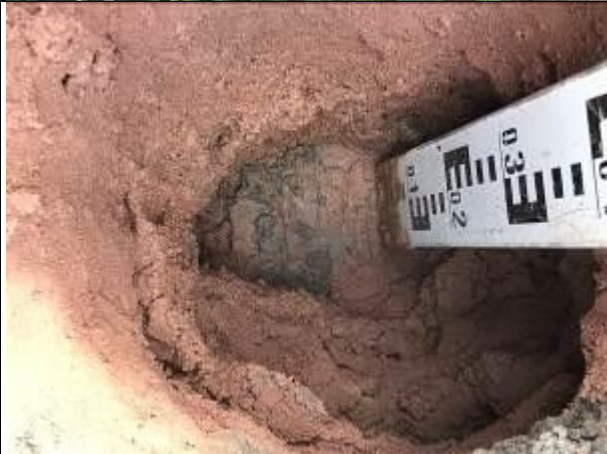
View of soil in capping layer excavation.
