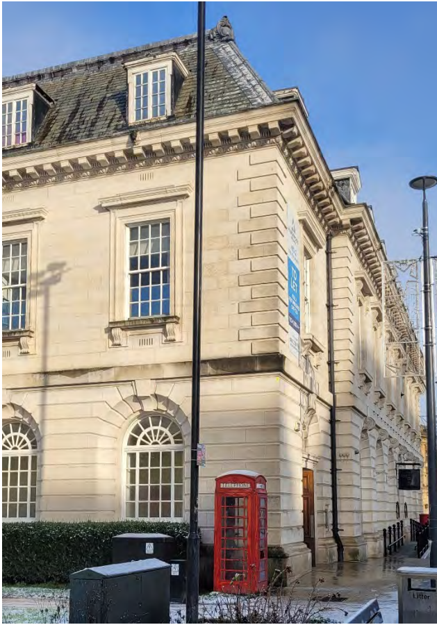
Plate 23 Old Post Office, looking north
