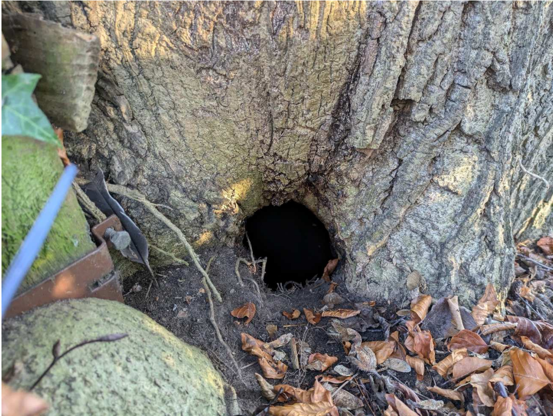
The cavity at the base of T20 which revealed a hollow stem and decay.
