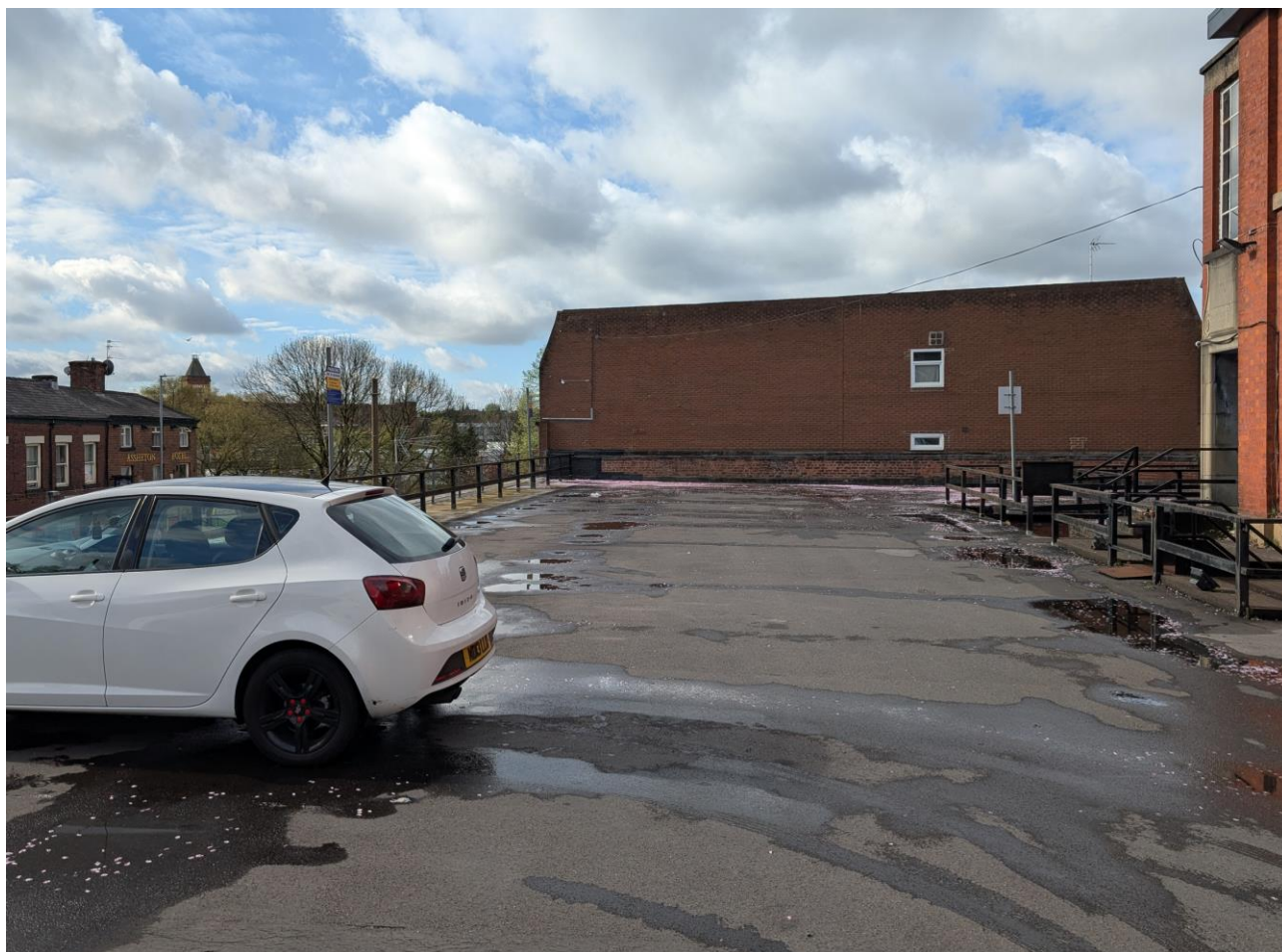
Figure 10: Tarmac hardstanding above undercroft retail units
