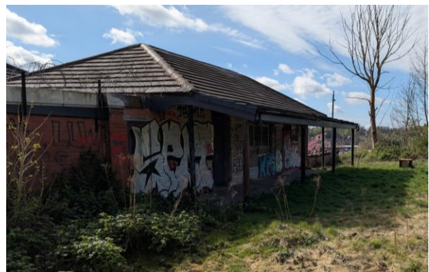
Figure 16: Western elevation seen from upper grass area
