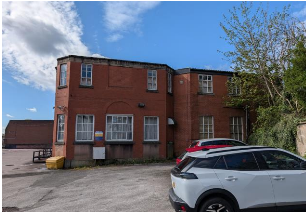
Figure 13: Northern elevation – extensions with flat roofs
