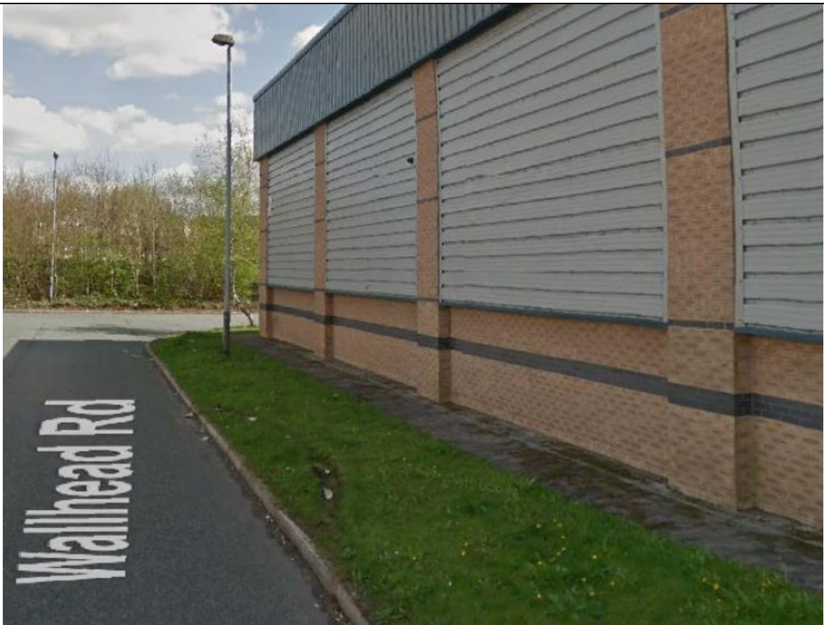
(Figure 11: This is the location of a previous approved application (Ref: 23/00071/TELE) that falls outside of the search area for this application but still carries valid precedent in sitting telecoms equipment within a business/retail park. Source: Planning Portal)
