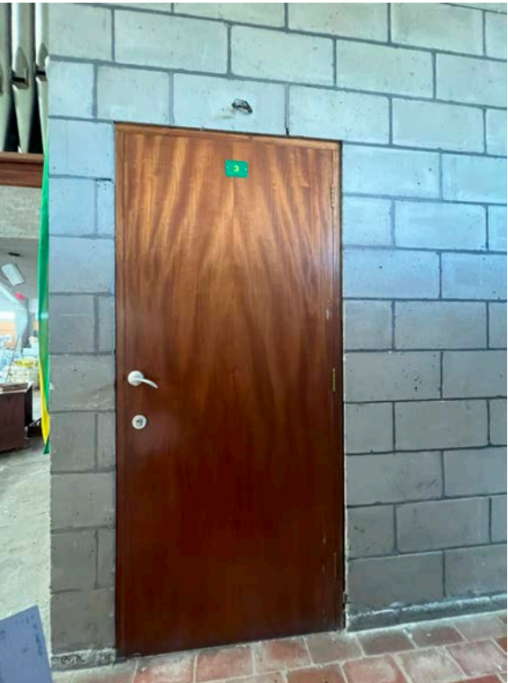
158 Internal Door to north of Sacristy
