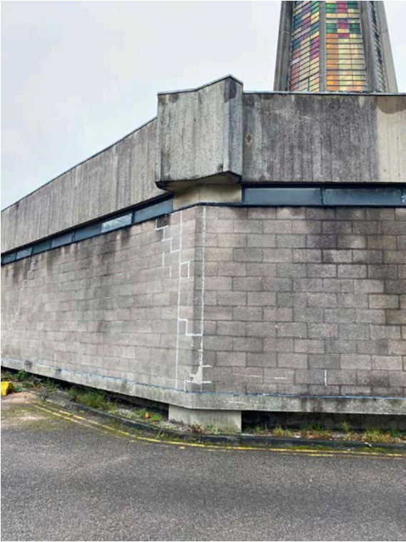
19 View of Concrete Structure
