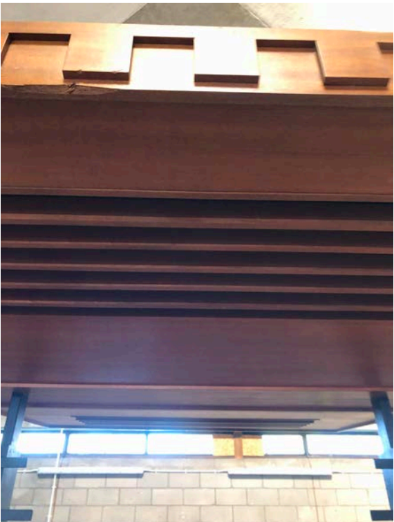
139 Detail of Ciborium to Blessed Sacrament Chapel
