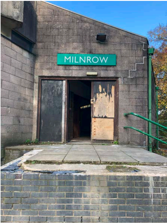
24 External Doors (South Entrance to Narthx)
