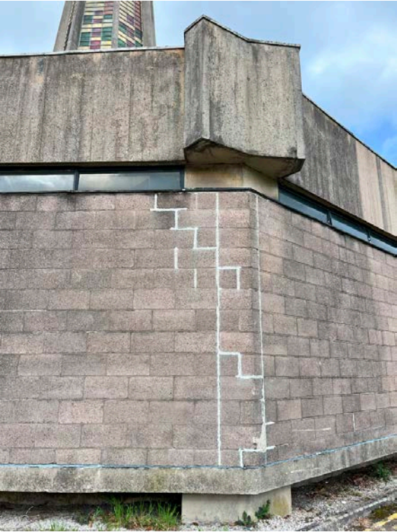
18 View of Concrete Structure
