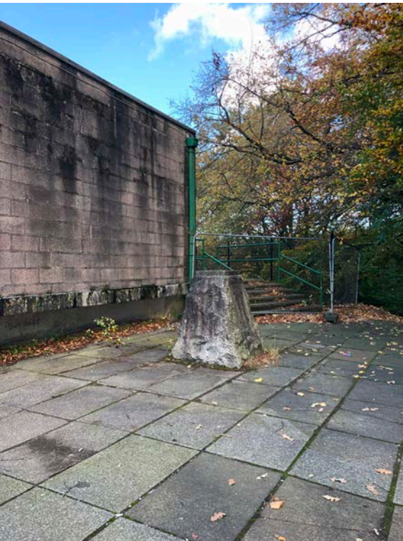
47 View of Paving to South of Narthex
