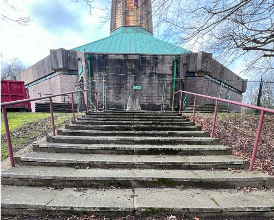
14 View of East Elevation looking Towards the Narthex
