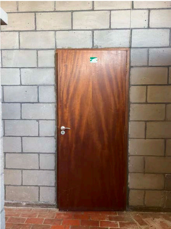
159 Internal Door to north of Sacristy
