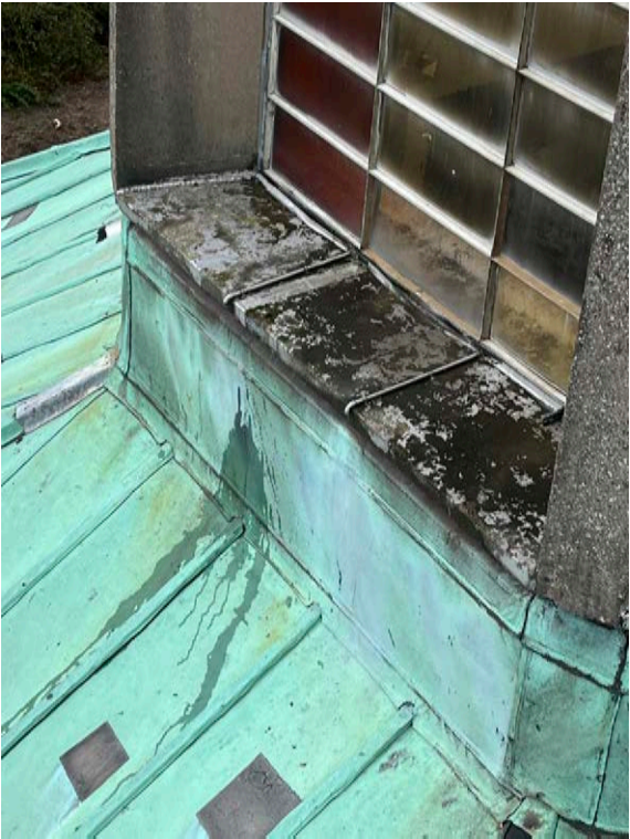
38 View of Base of Glazed Lantern
