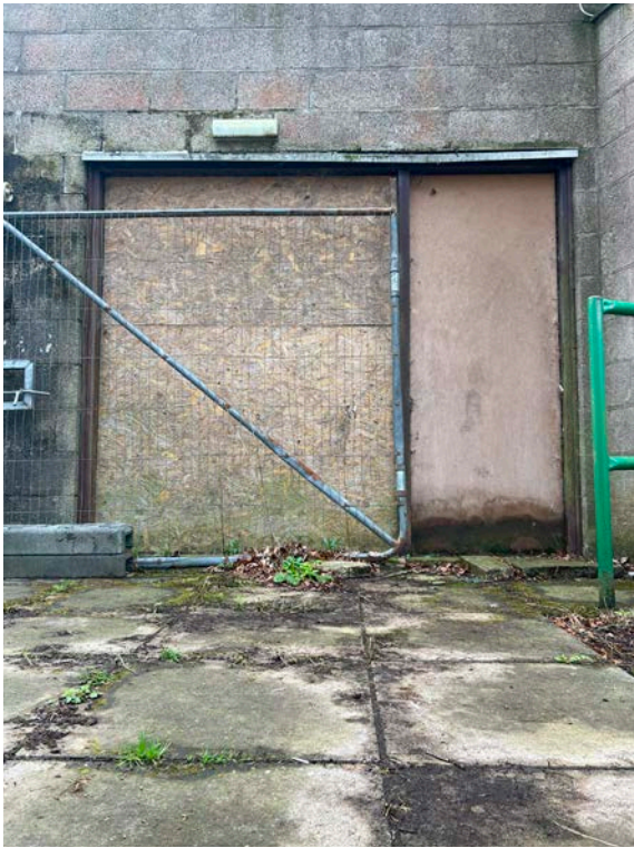
25 External Doors (North Entrance to Narthex)
