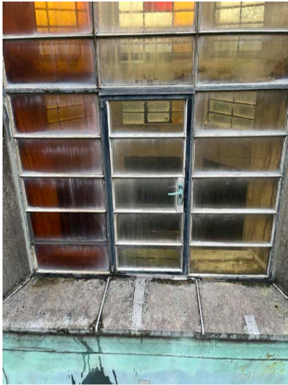
40 Detail of Glazed Lantern
