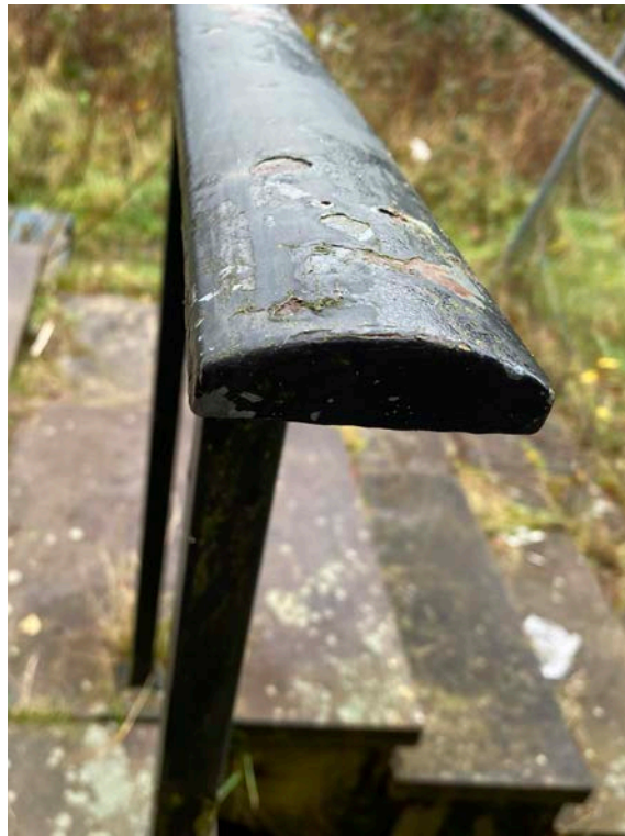
50 Detail of Handrail to West Porch Steps
