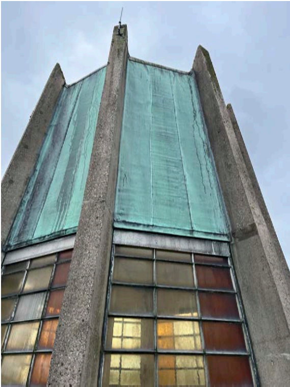
37 View of Glazed Lantern
