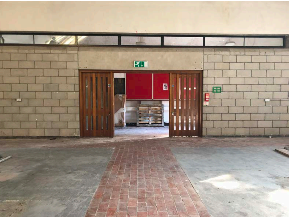
160 Internal Clerestory Windows viewed from within Chapel
