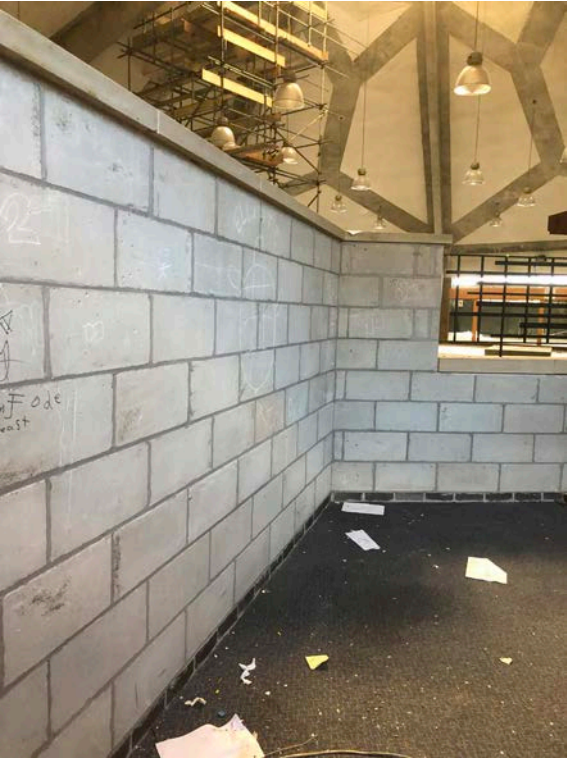
140 View of Walls enclosing Blessed Sacrament Chapel
