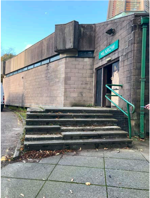
15 View of South Elevation looking Towards the Narthex
