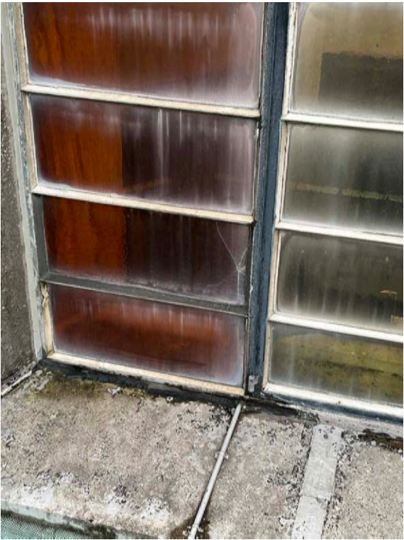
42 Detail of Glazed Lantern
