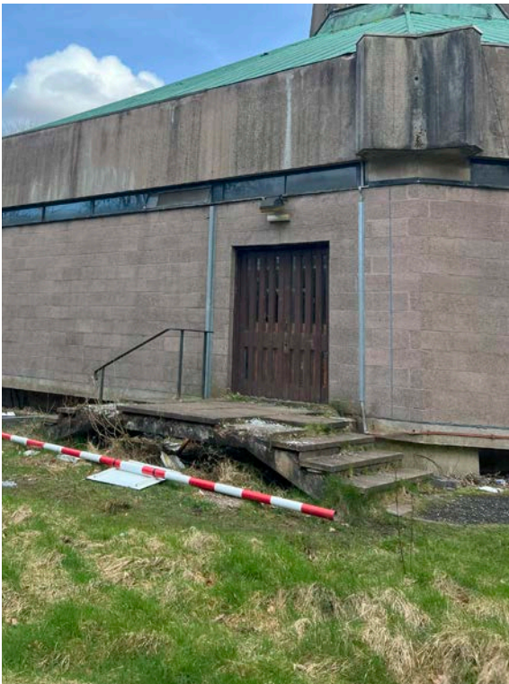
48 View of Steps to West Porch
