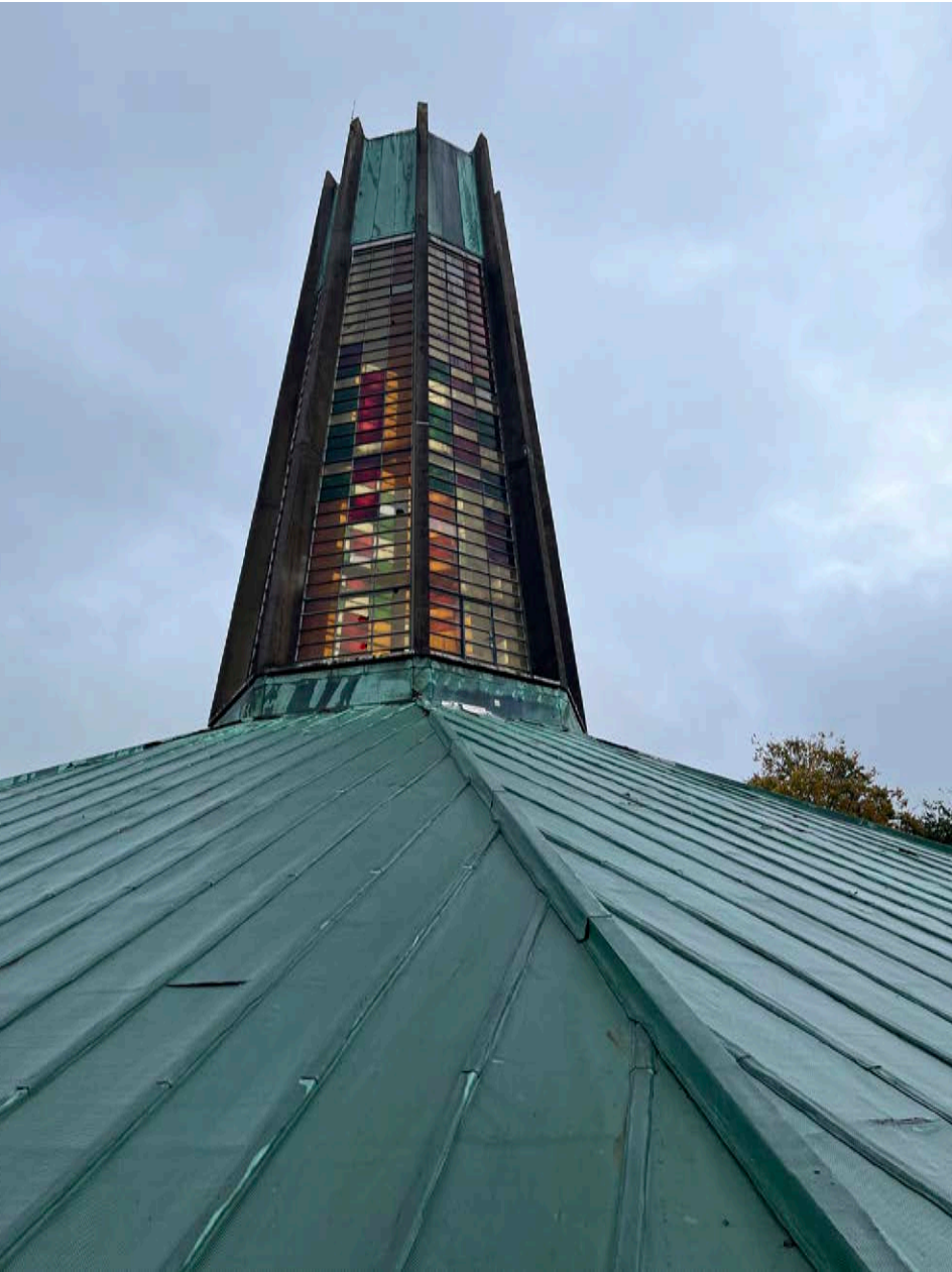
30 View of Copper Faced Roof and Glazed Lantern
