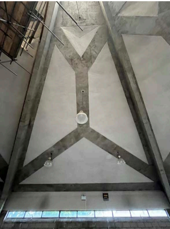
166 View of Soffit
