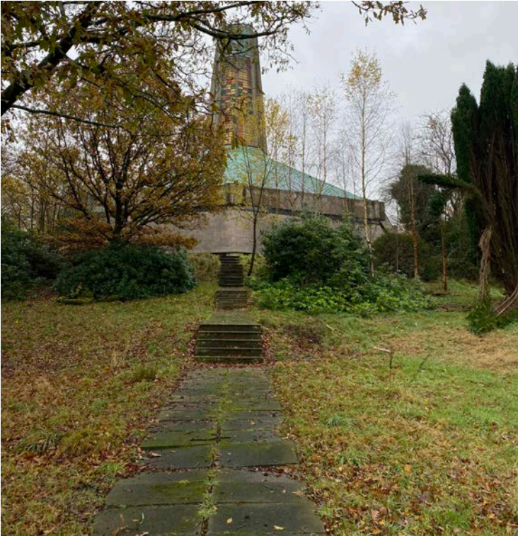
3 View from the Existing Stepped Access towards the building from the North
