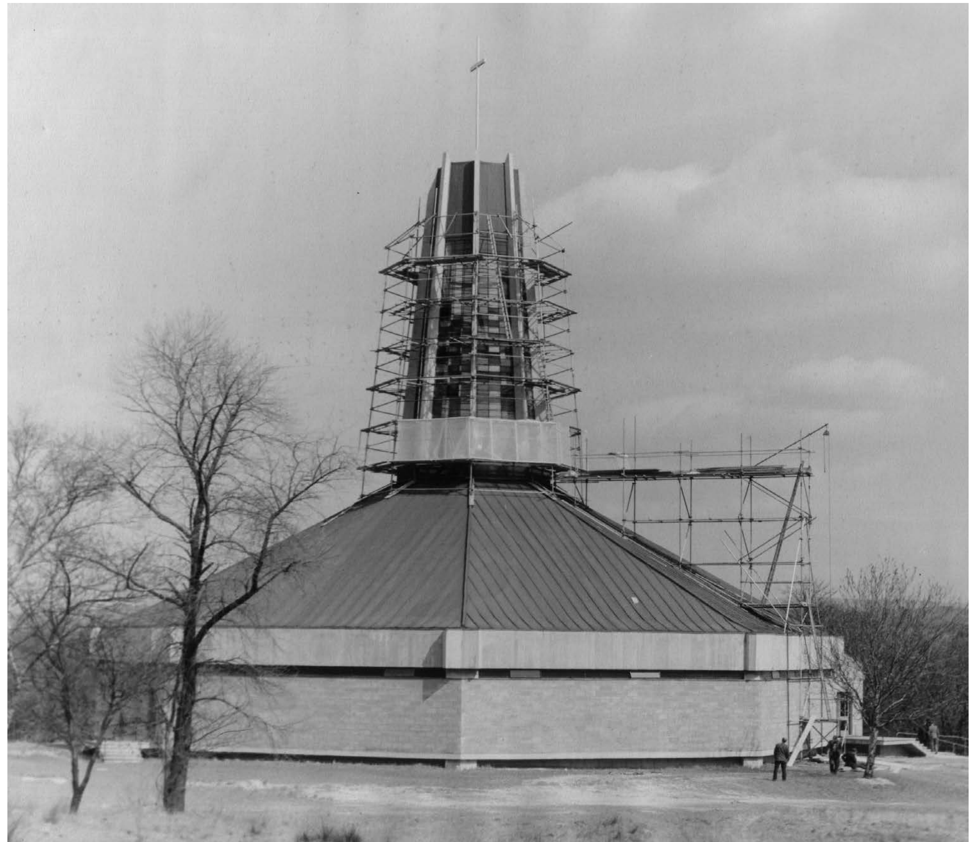
Figure 4.24 The Chapel during construction (Source: Rochdale Archives)
