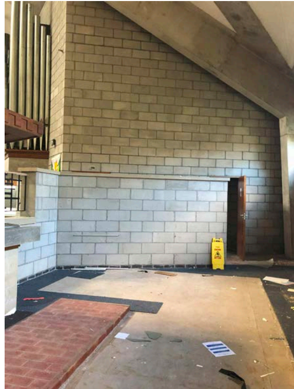
117 View from within Blessed Sacrament Chapel
