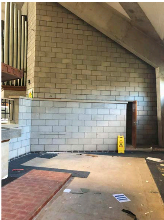
143 View of Walls enclosing Blessed Sacrament Chapel
