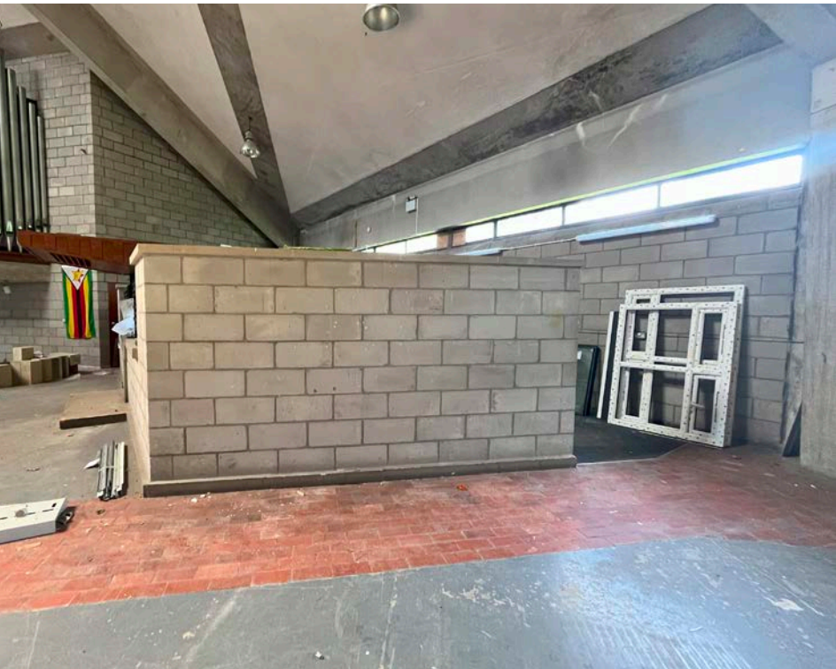
136 View of Walls enclosing Blessed Sacrament Chapel
