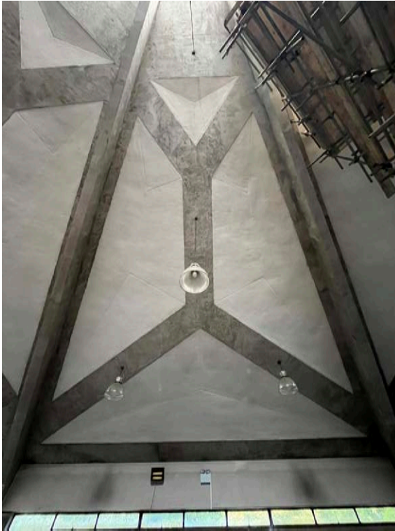
164 View of Soffit
