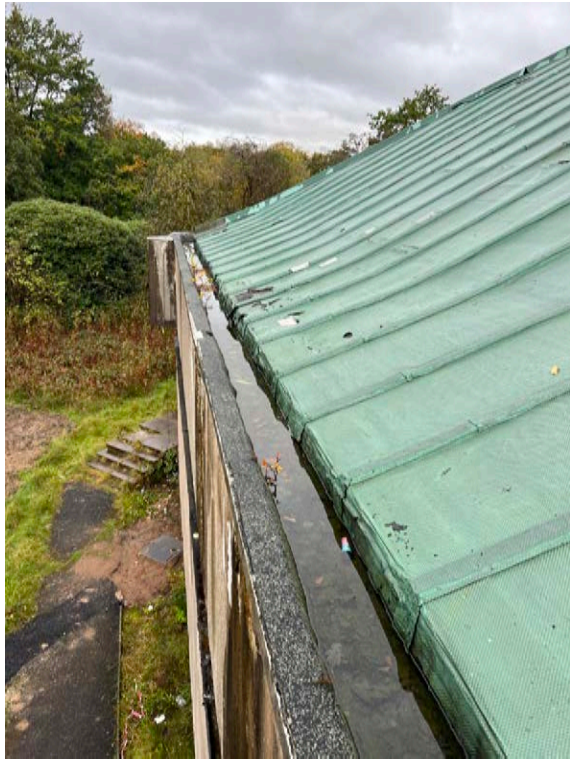
31 Parapet Gutter Detail
