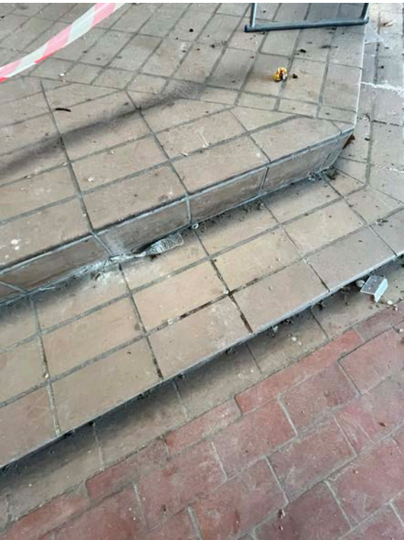
124 View of steps to Sanctuary raised Dias
