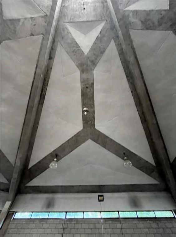
163 View of Soffit
