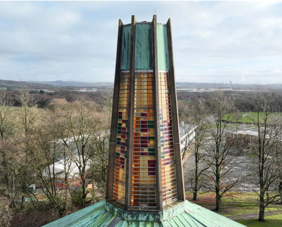
35 View of Glazed Lantern Image credit - Castle Keep Surveys
