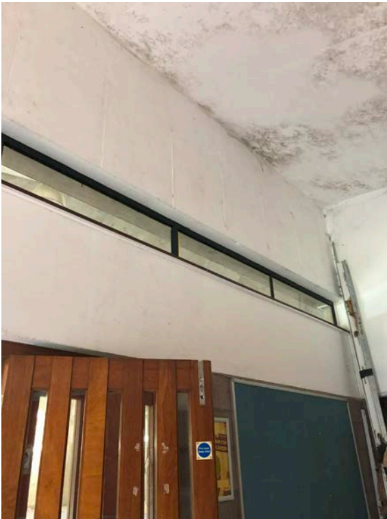
161 Internal Clerestory Windows viewed from within Narthex
