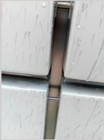
Photograph 16: External metal cladding, block A and block B
