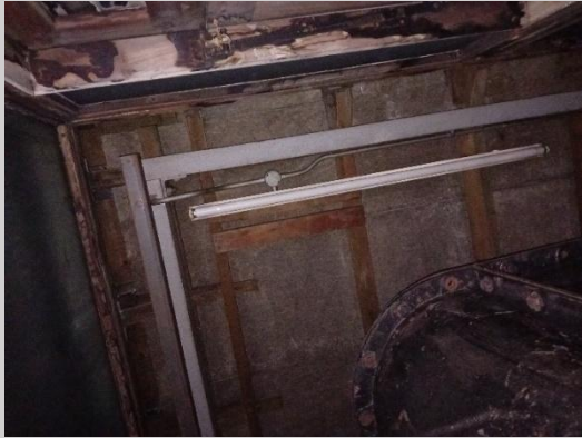
Photograph 20: Water tank room, block B
