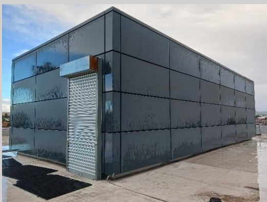
Photograph 24: Metal clad buildings on top of flat roofs.
