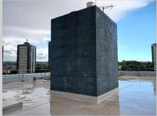
Photograph 21: Brick structure on roof of block B. Only accessible externally.
