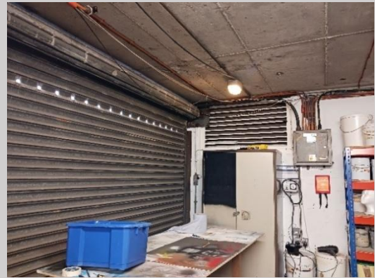
Photograph 27: Garages, potential access for bats.
