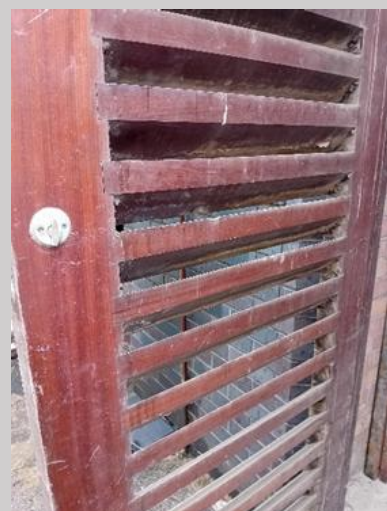
Photograph 25: Slatted door garages
