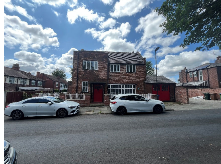
Plate 30: North (front) elevation of Arkholme.
