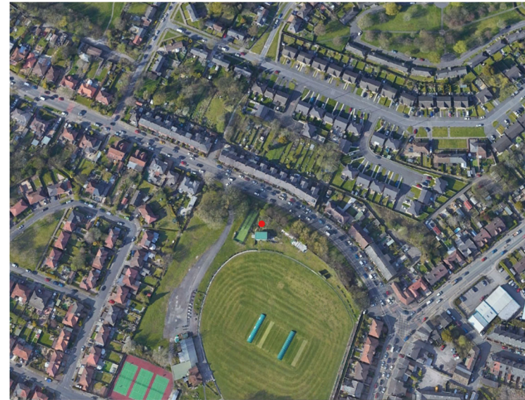
Plate 4: Aerial photograph of the Site (as indicated by the red dot) and its immediate surrounds.
