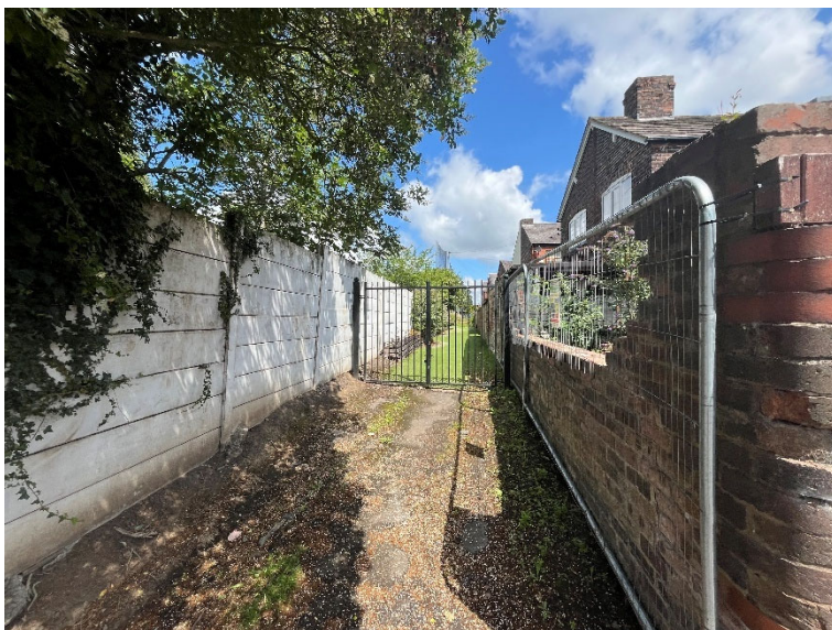
Plate 29: Rear lane behind Nos. 51 and 53 Rochdale Road.
