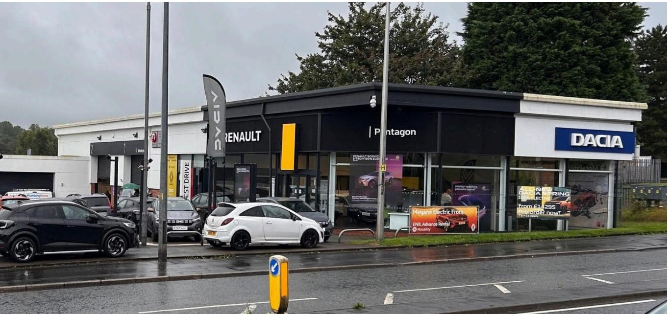
Site looking at the main facade from Queensway
