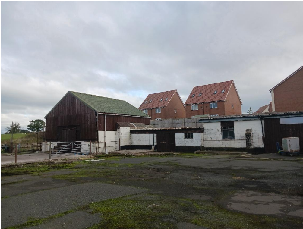
View of existing buildings on the site and adjacent housing located to the east.
