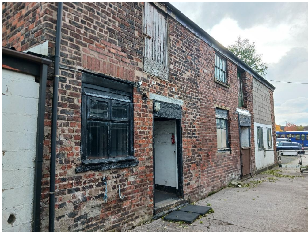
View of existing buildings on the site.
