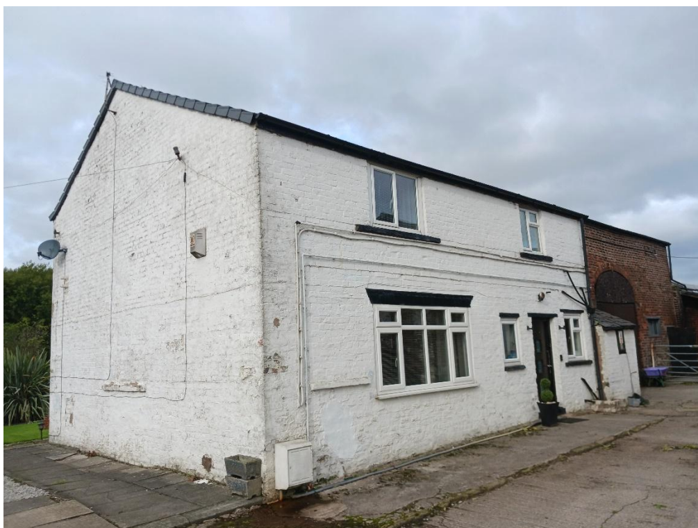
View of existing buildings on the site.
