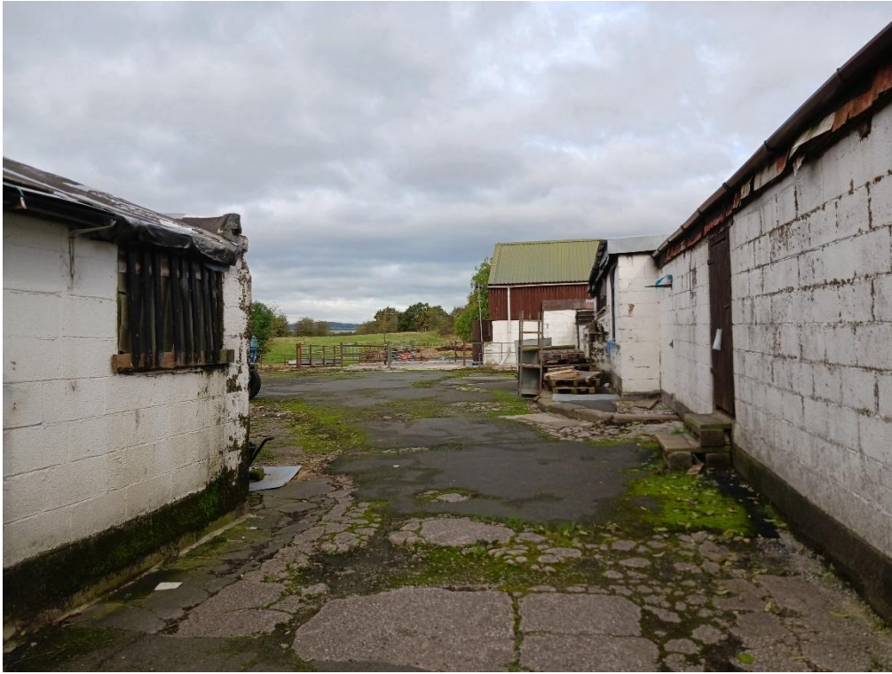
View looking between the existing site buildings looking north.
