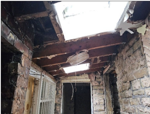
Figure 12: Second floor, exposed roof void above
