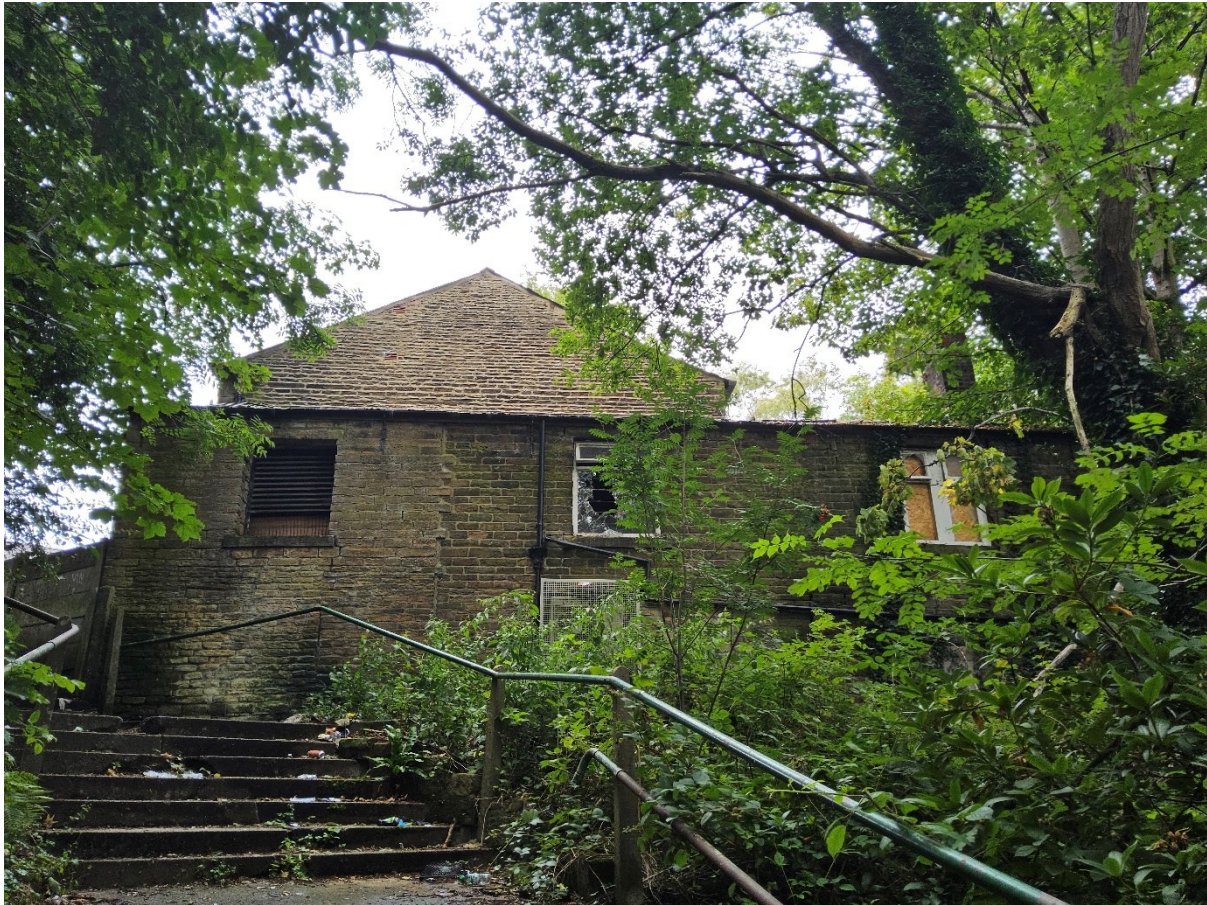
Figure 14: Scrub and scattered trees to east of building
