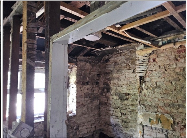
Figure 11: Exposed roof void from second floor
