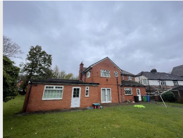
Photograph 2- Southern aspect of the building
