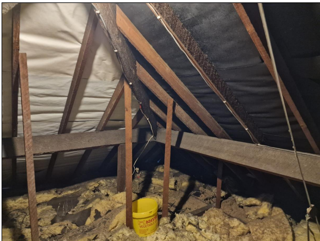
Plate 6 – General character of the internal loft void (L1)
