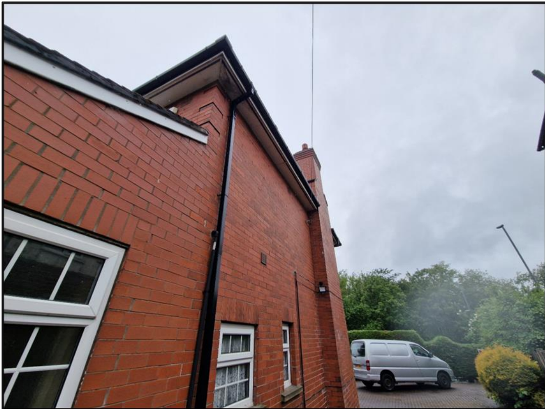
Plate 8 – The general character of the sealed UPVC soffit boxes around the building
