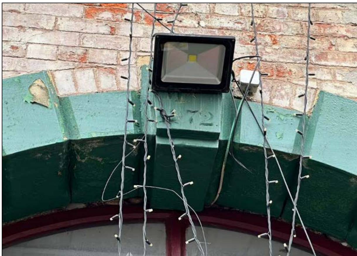
4. The date of 1872 on the archway keystone
