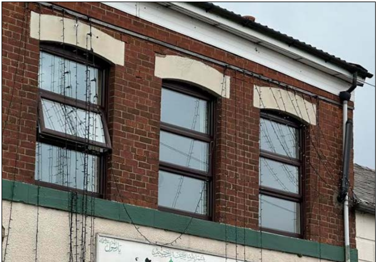
5. Windows all have replacement framing
