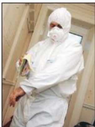
Cleaning with damp rag using patting action
