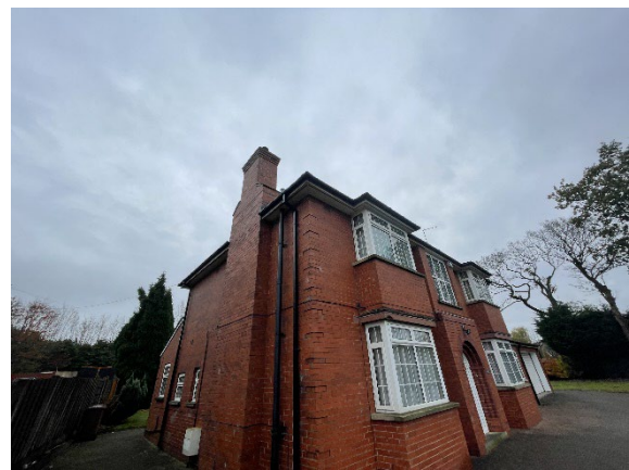
Photograph 4- Western aspect of the building with view of the chimney
