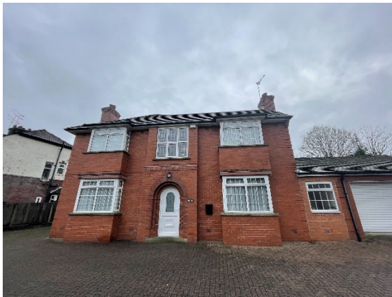
Photograph 1- Northern aspect of the building
