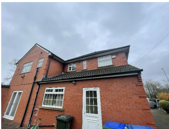
Photograph 3- Southern aspect of the building with view of the second floor
