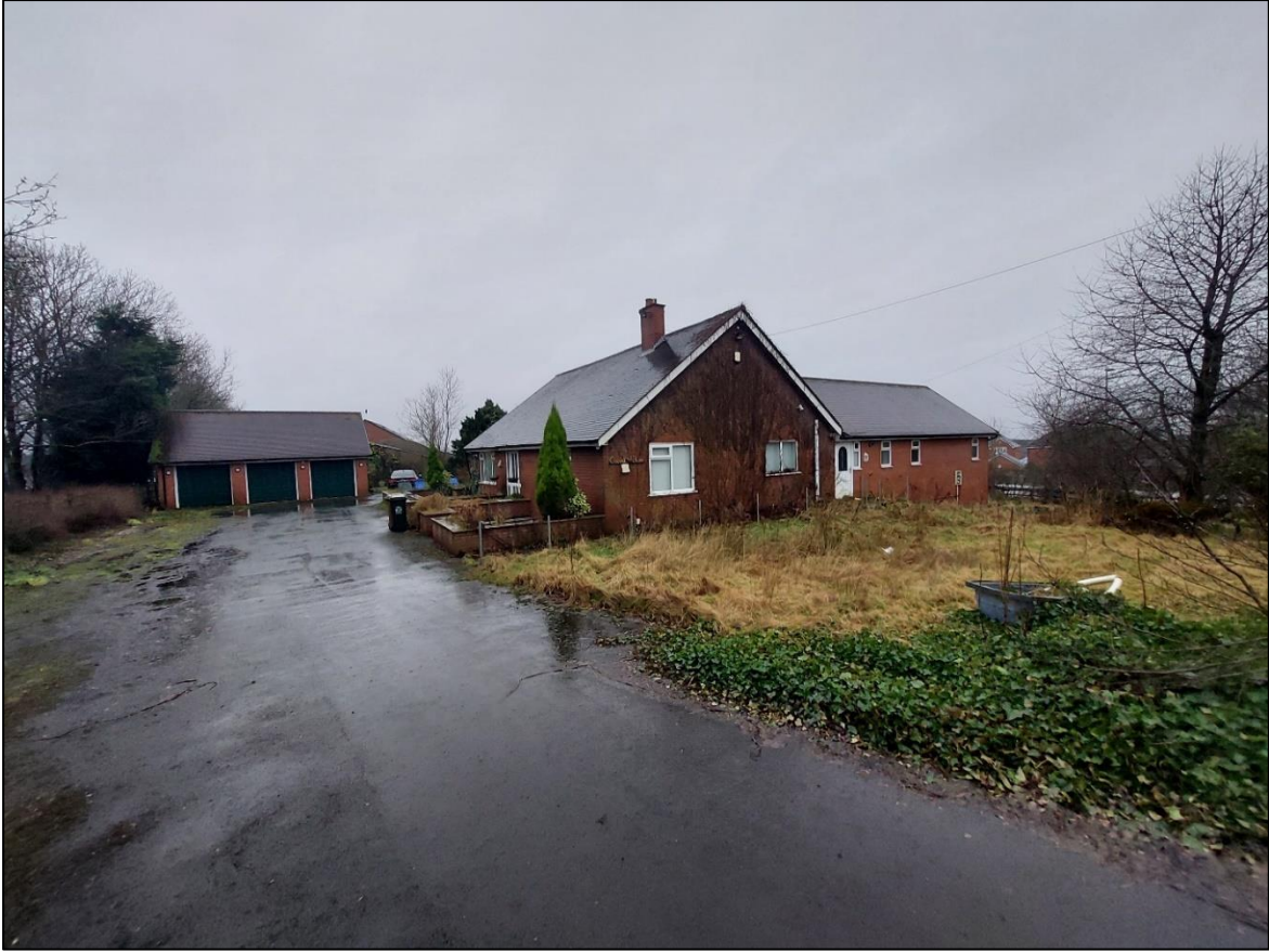
View from Existing Site Access of Dwelling and Garage (Facing West)
