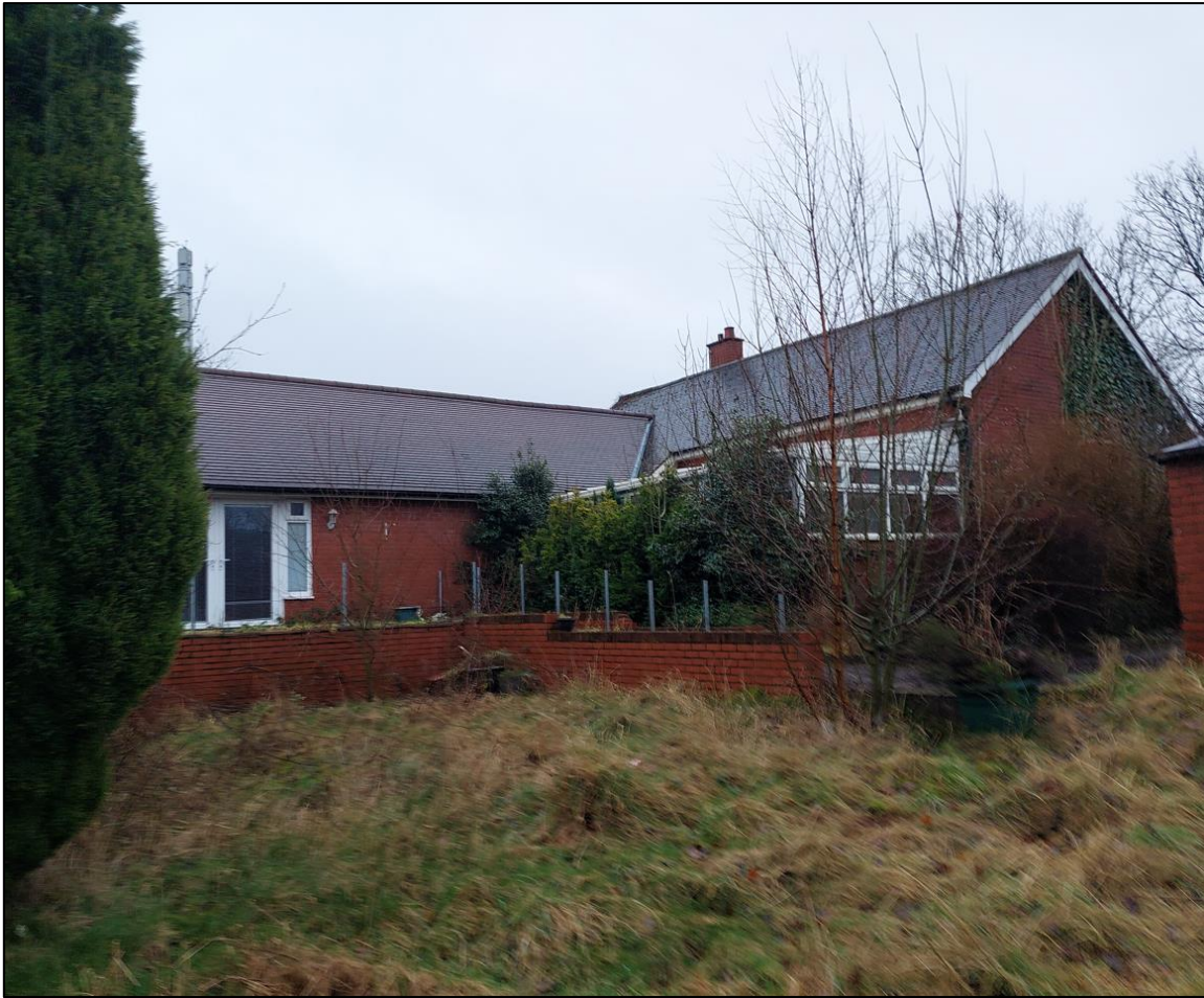
View of Dwelling (Facing South East)
