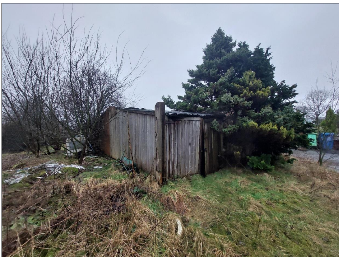
View of Dilapidated Outbuilding (Facing North East)
