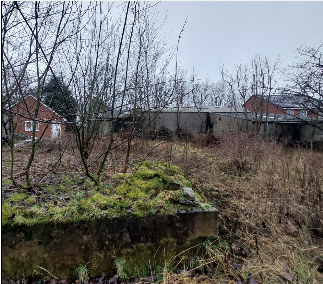
View of Garage and Dilapidated Former Agricultural Building (Facing South)
